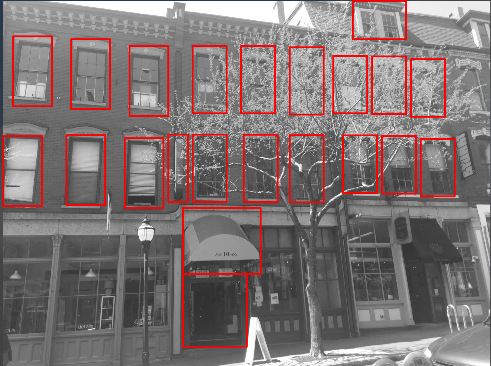
10 Exchange Street – Exchange Street Proposed Demo/Upgrade
