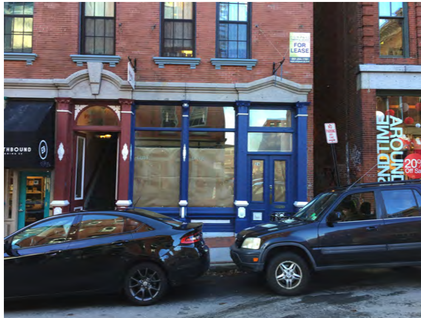
Exchange St. (NE) Elevation
