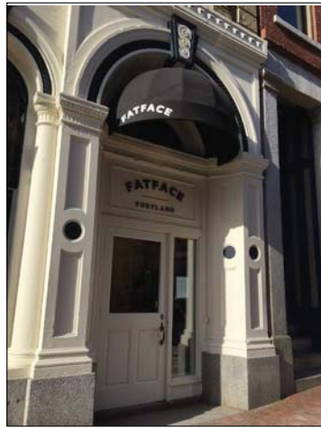
existing shop front
