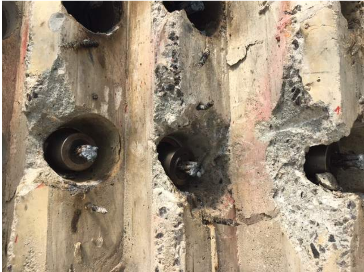
Photo 1: Barrels installed at the anchors of the PT strands
