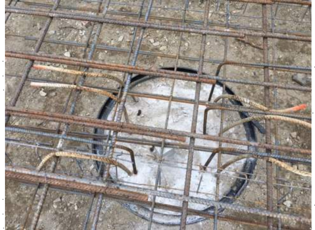
Photo 2: Four replaced dowels at pier
