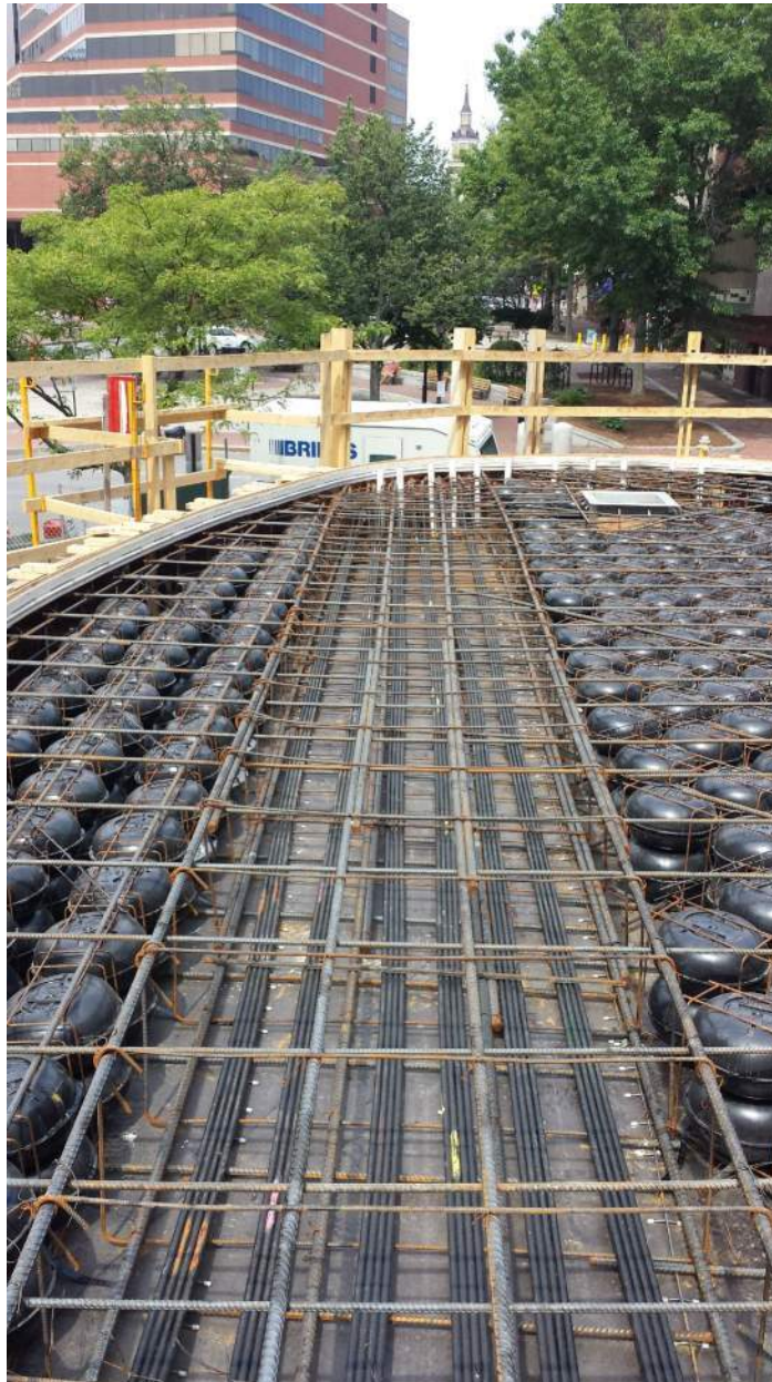
Photo 1 – Straightened Tendons in Beam 1
