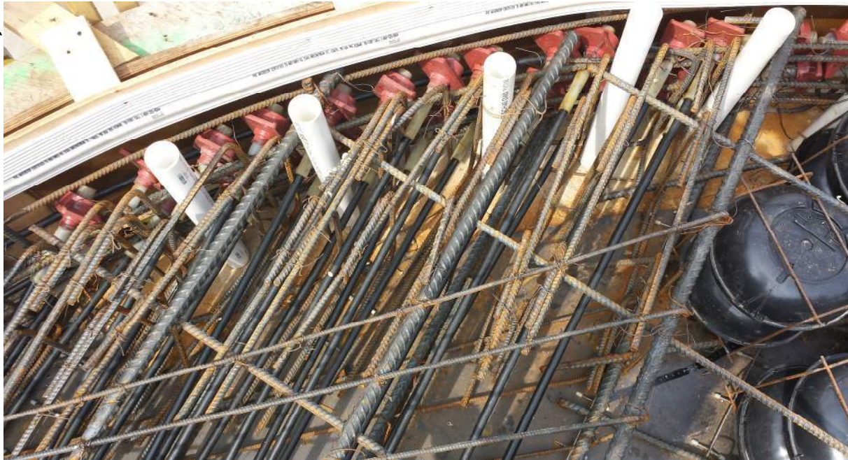
Photo 2 – Hairpins Straightened to Vertical
