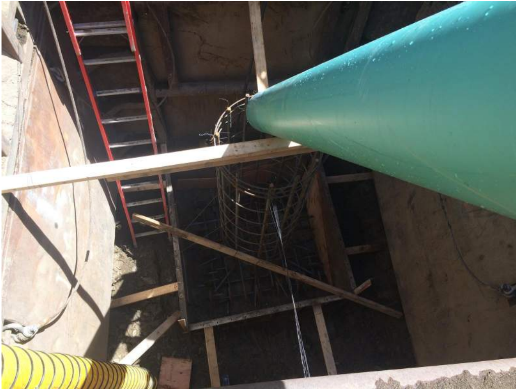
Photo 1: Preplacement view of footing.
