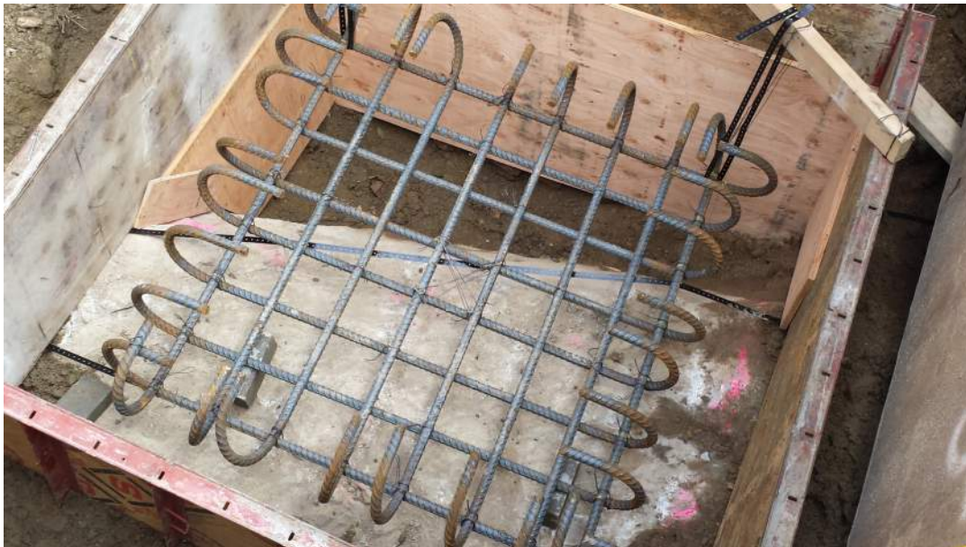
Photo 1: Steep Drop in Ledge Profile at Footing Near WP-4
