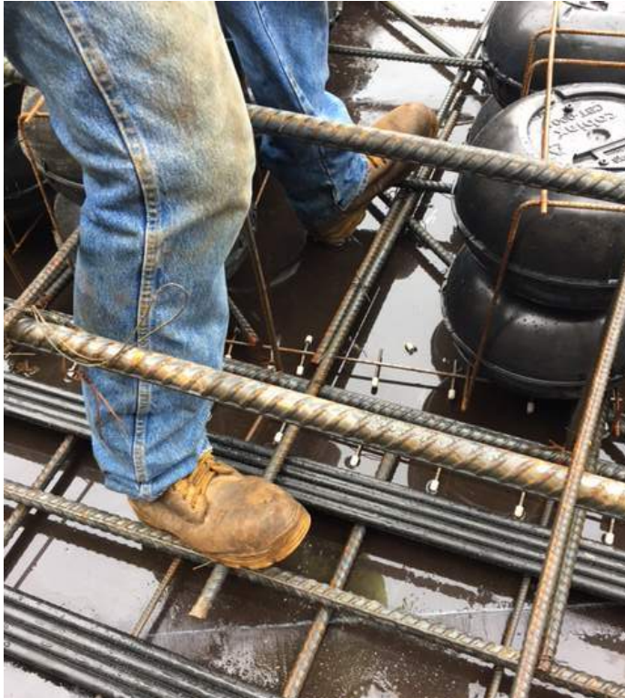
Photo 2 – Lapped Bars Added to Extended into Beam
