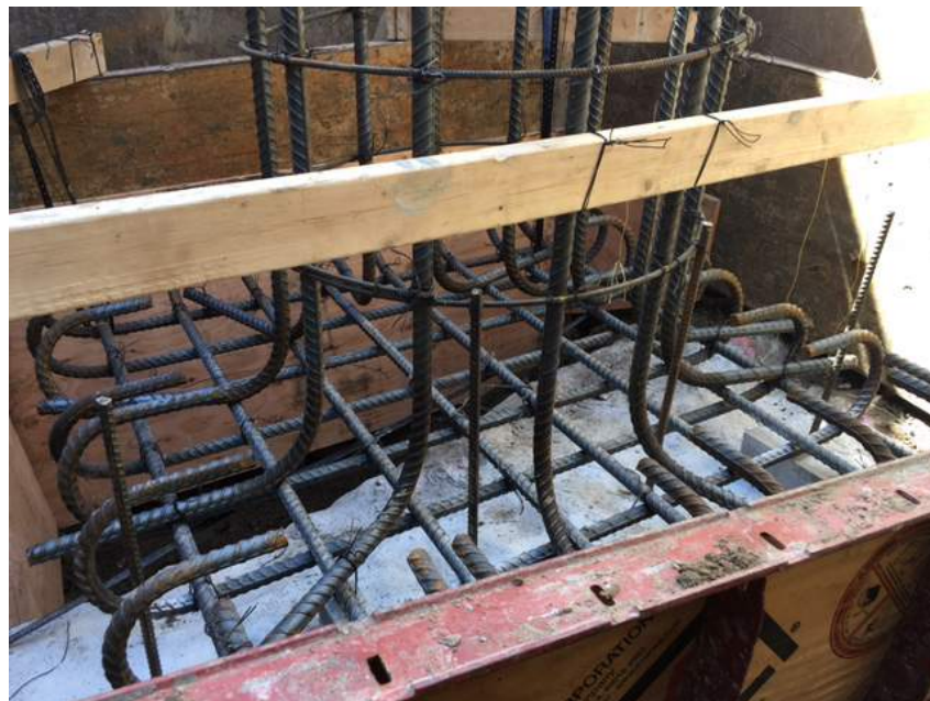
Photo 2: Vertical Pins Added to Stabilize Footing on Uneven Ledge
