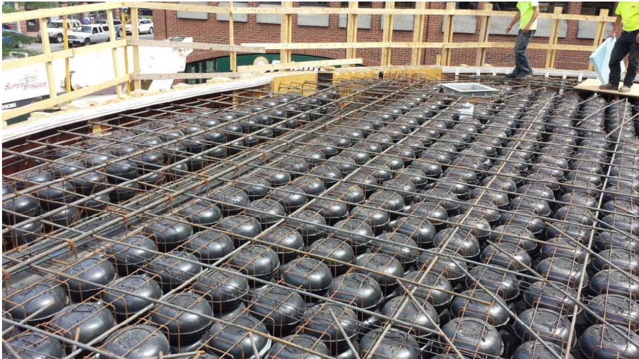
Photo 3 – Void formers positioned with the correct spacing
