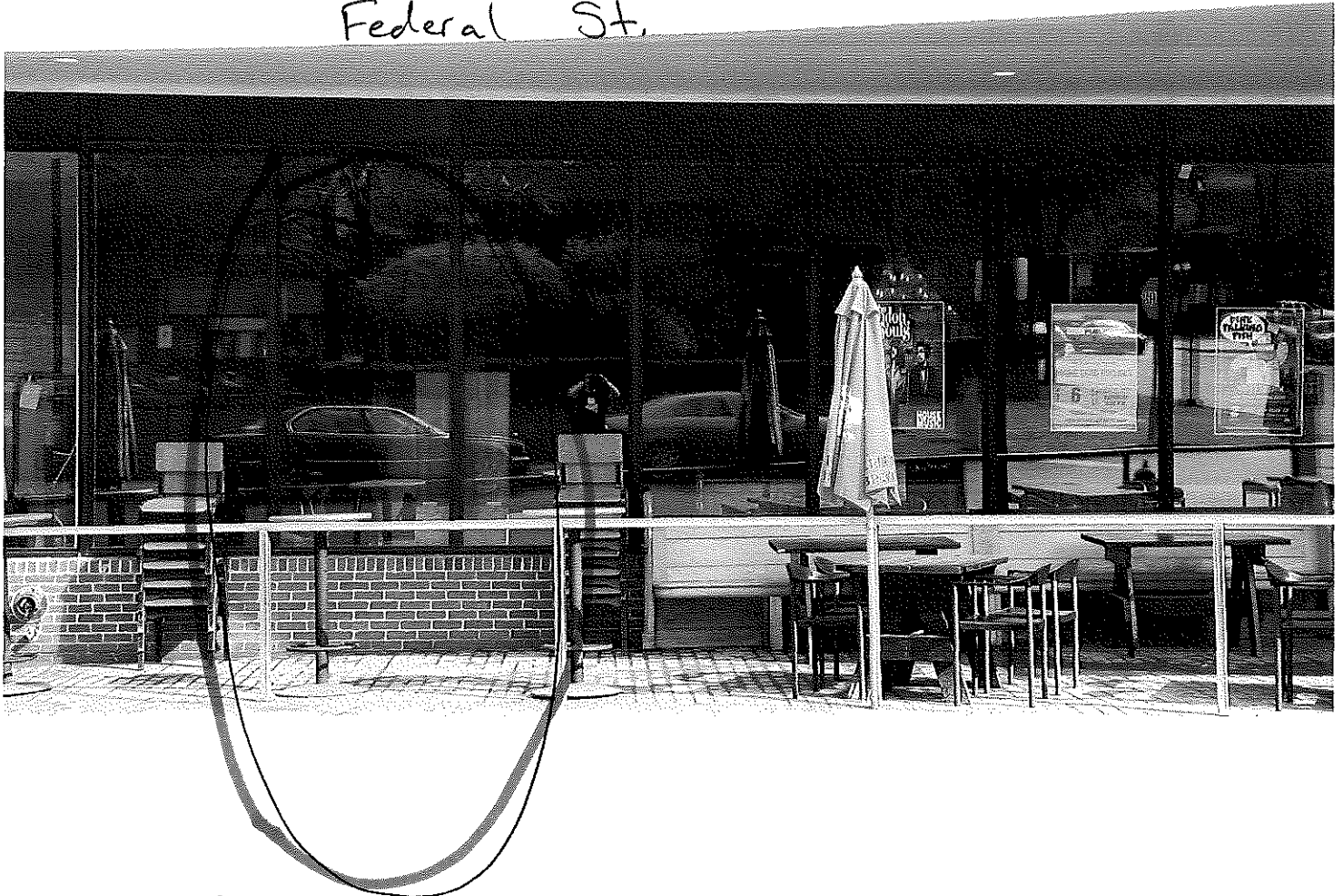
front view - window installation site
