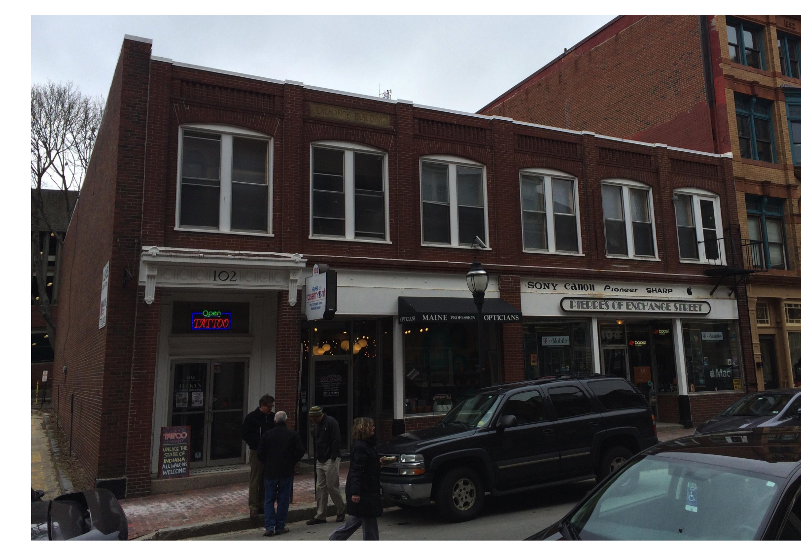
102 EXCHANGE: EXISTING EXTERIOR
