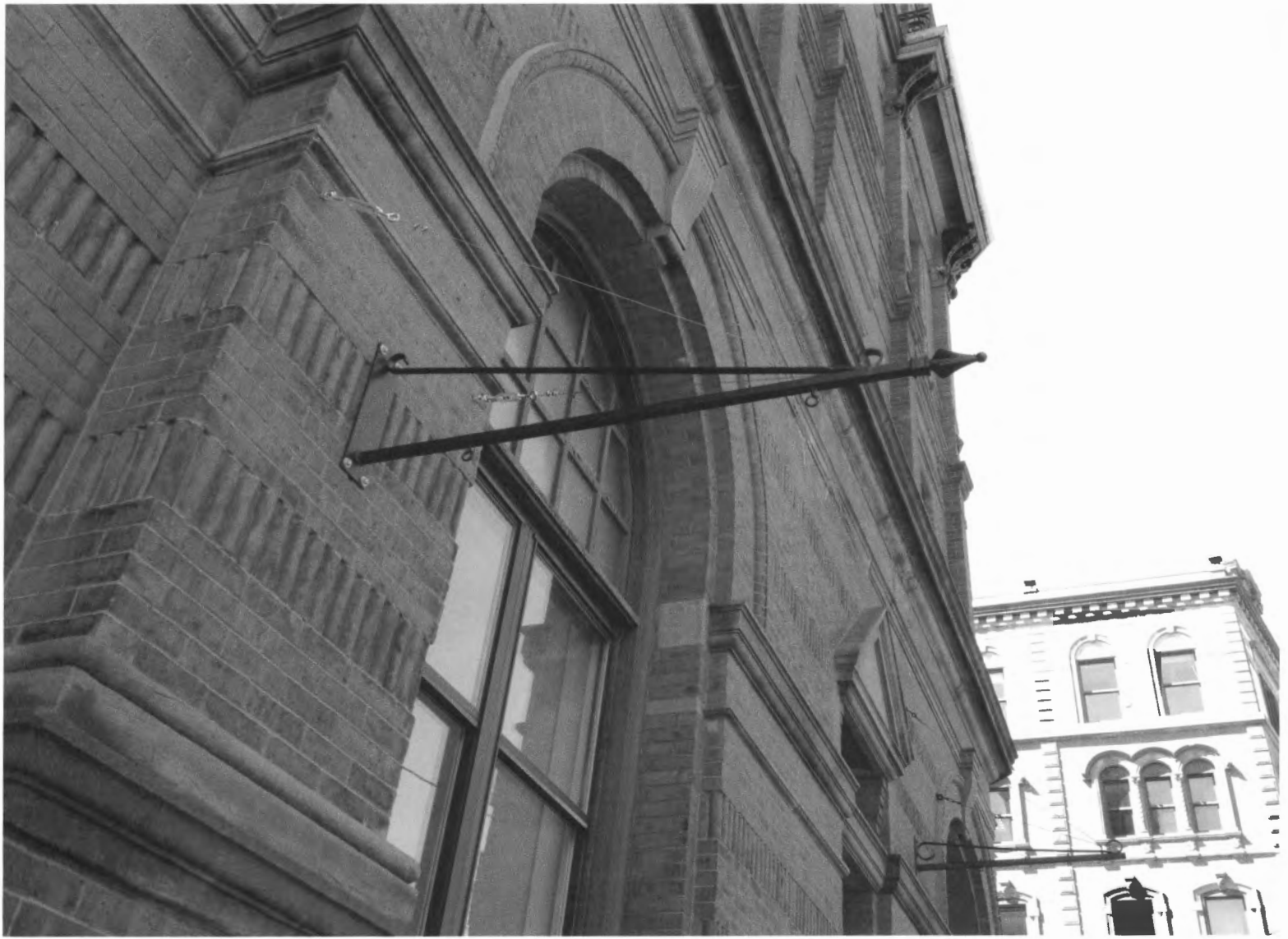
EXISTING BRACKET w/ CABLES (10' 4" ABOVE SIDEWALK)
