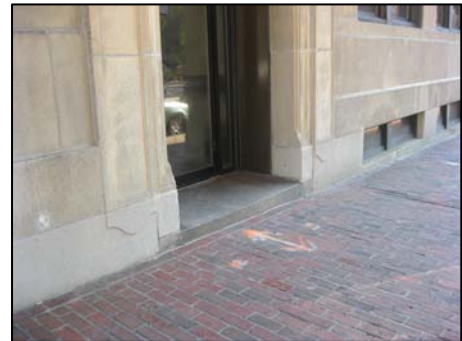
Figure 1 – Existing Exchange Street Entrance
