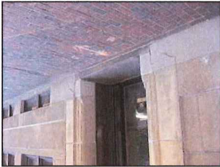
Figure 1 – Existing Exchange Street Entrance
