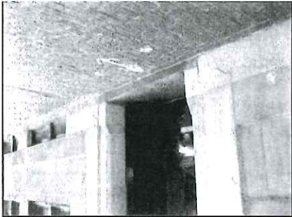
Figure 1 – Existing Exchange Street Entrance
