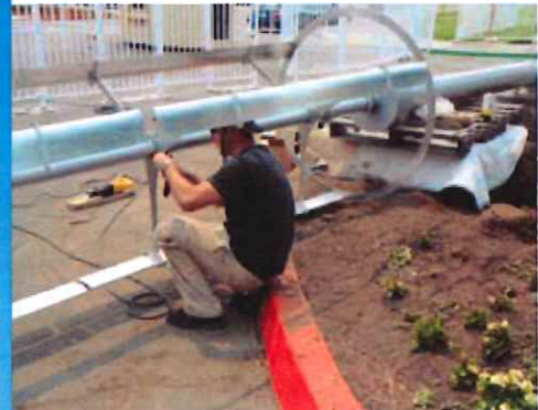
4. Assemble Rotor
