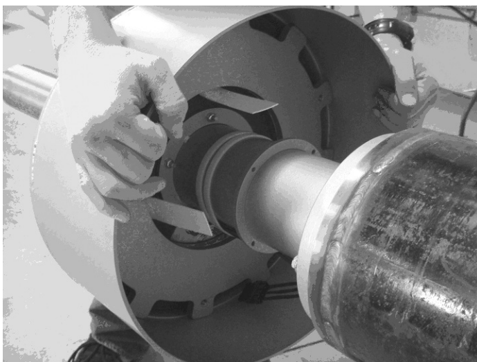
Figure 2-37: Pulling the Generator Housing towards the Top of Bottom Shaft
