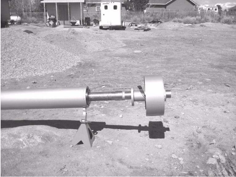
Figure 2-30: Resting the Generator over the Bottom Shaft
