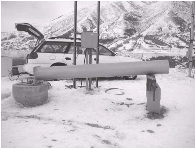
Figure 2-13: Resting the Base Pole on a Sturdy Support
