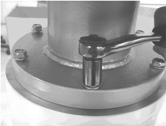
Figure 2-33: Securing the Generator to the Top of the Base Pole
