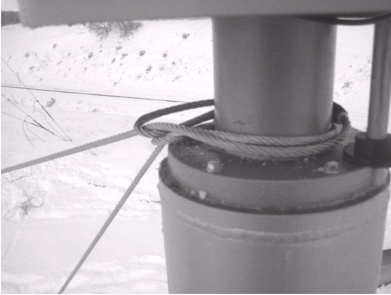
Figure 2-70: Wrapping the Gin Pole Cable Around the Armature Tube
