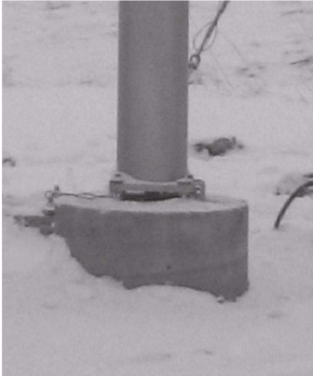
Figure 2-74: Top Hinge Plate Tightened to the Foundation Rods
