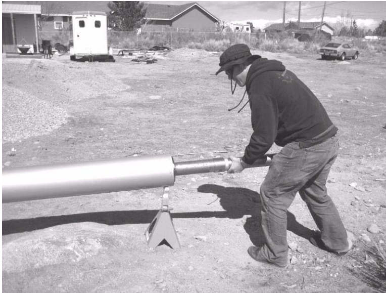
Figure 2-24: Inserting the Bottom Shaft Partially into the Base Pole
