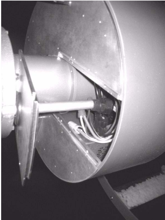
Figure 2-51: Connecting Wires Through the Base Pole
