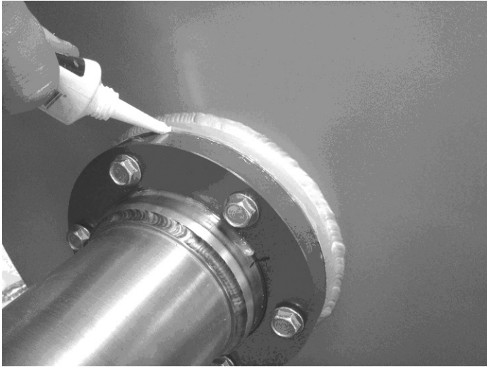
Figure 2-40: Sealing Interface Between the Bottom Shaft and Generator Clamp
