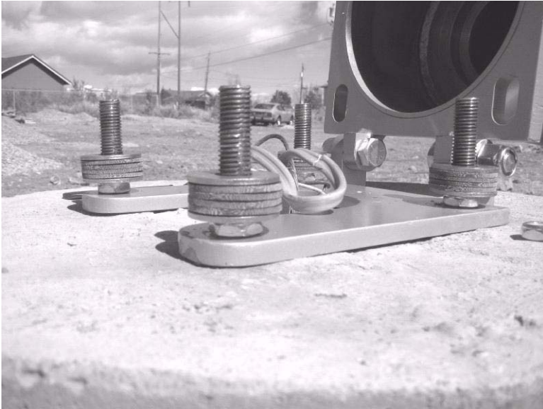
Figure 2-14: Washers Installed on the Bottom Hinge Plate
