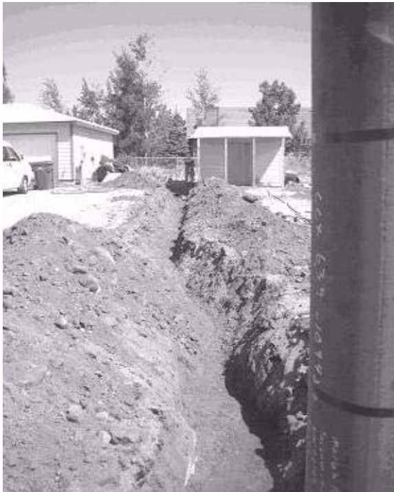
Figure 2-14: Trench for Conduit
