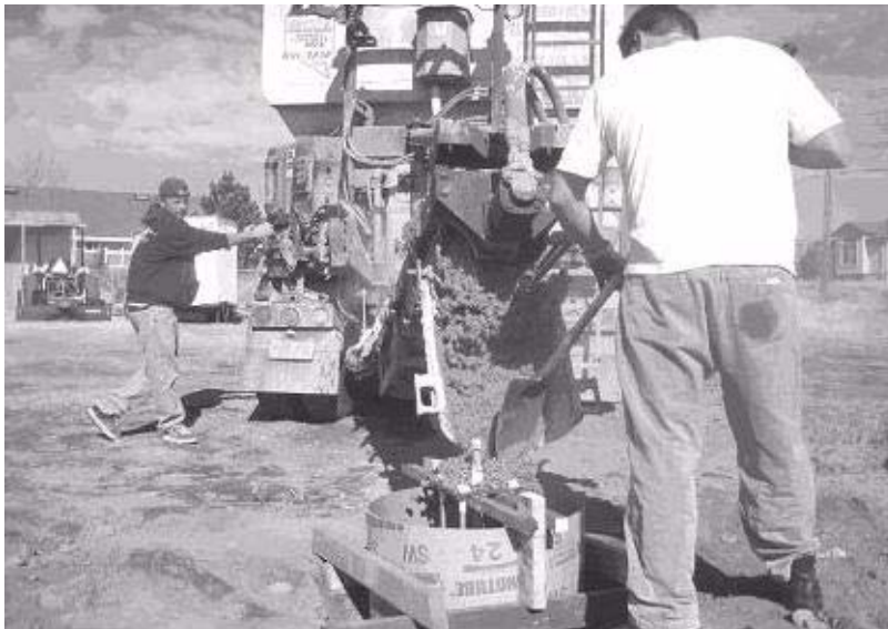
Figure 2-11: Pouring the Concrete
