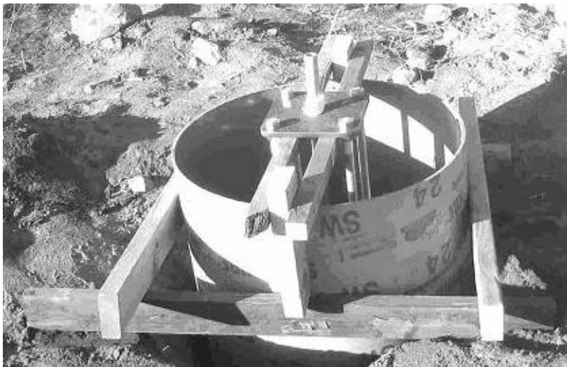
Figure 2-9: Foundation Template Installed in the Foundation Tube
