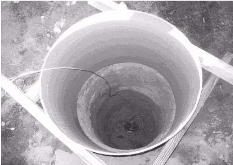
Figure 2-8: Ground Wire Attached to Grounding Plate in Foundation Hole
