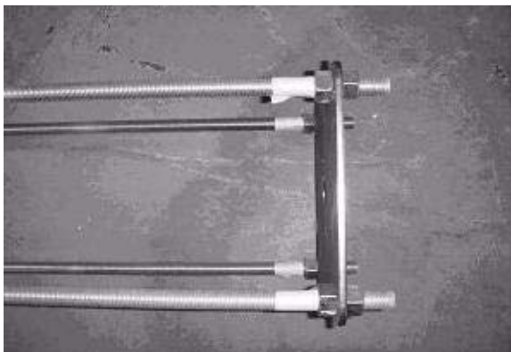
Figure 2-7: Protecting Foundation Rod Threads with Tape
