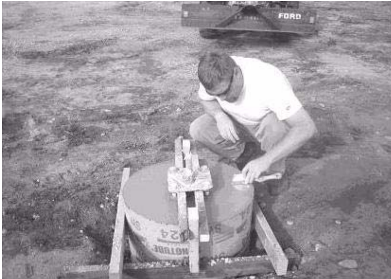
Figure 2-12: Leveling the Concrete to Be Even with the Sonotube
