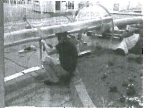
4. Assemble Rotor
