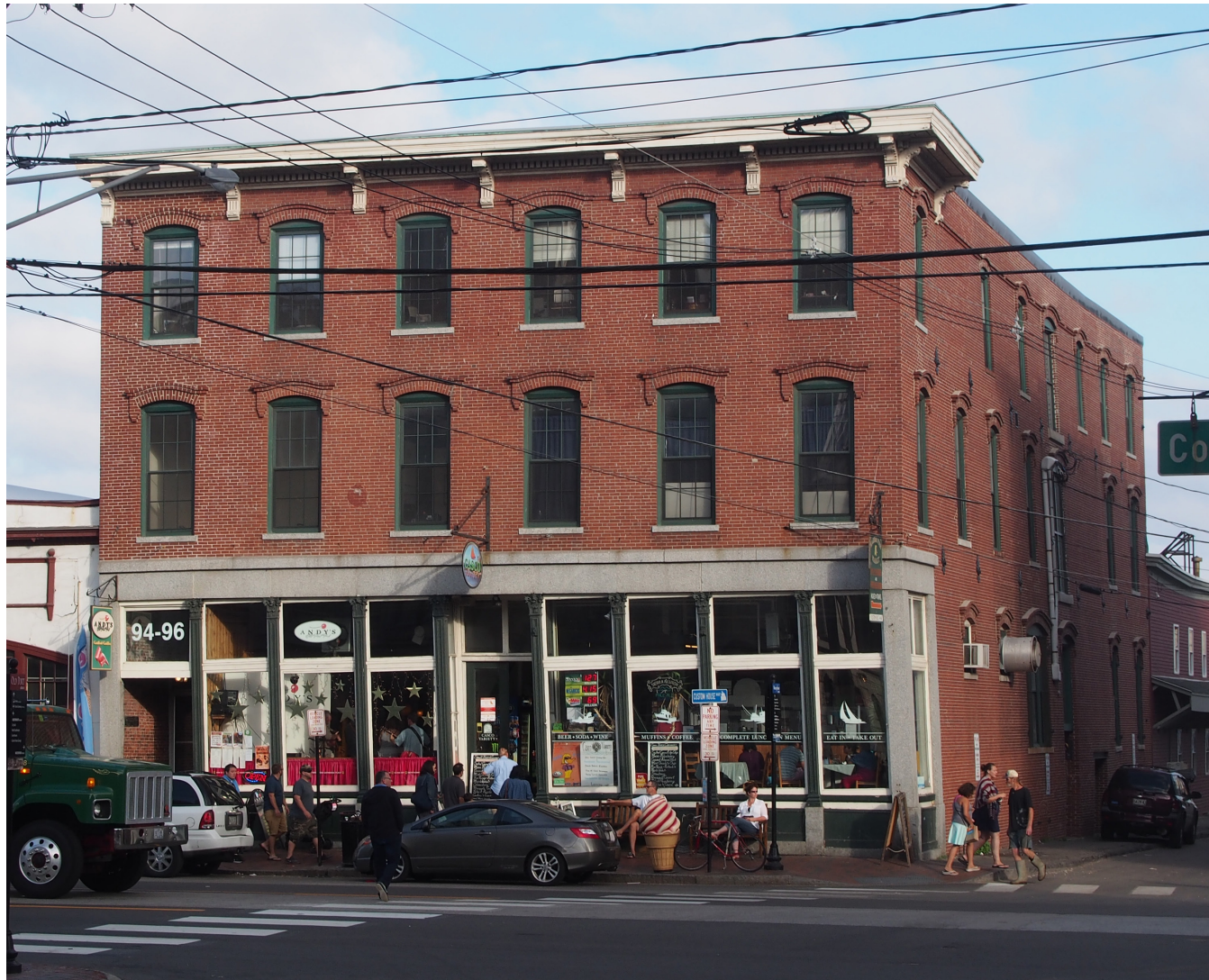
92-96 Commercial Street, existing conditions
