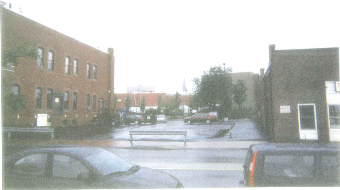
LOOKING NORTHERLY SHOWING ENTRANCE FROM COMMERCIAL ST.
