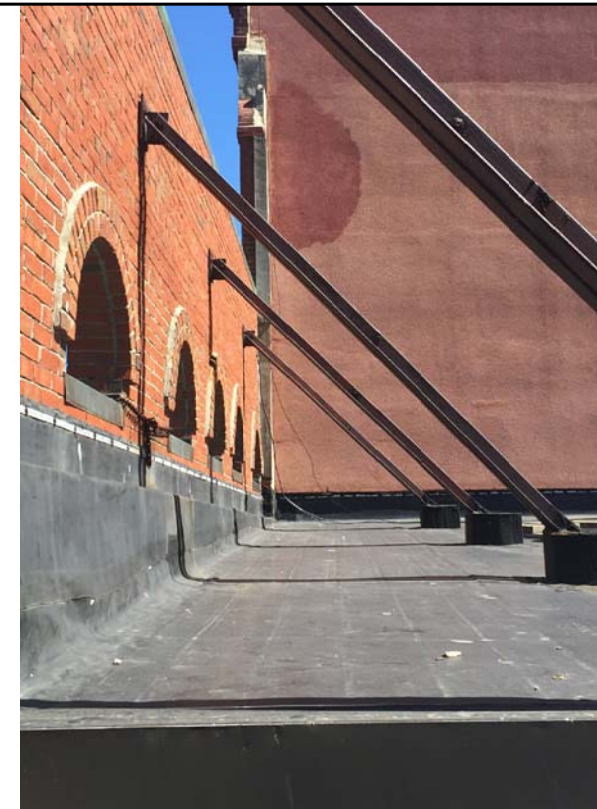
4 EX. PARAPET SUPPORT SCALE: NTS
