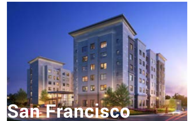
San Francisco Residence Inn Walnut Creek; Walnut Creek, CA
