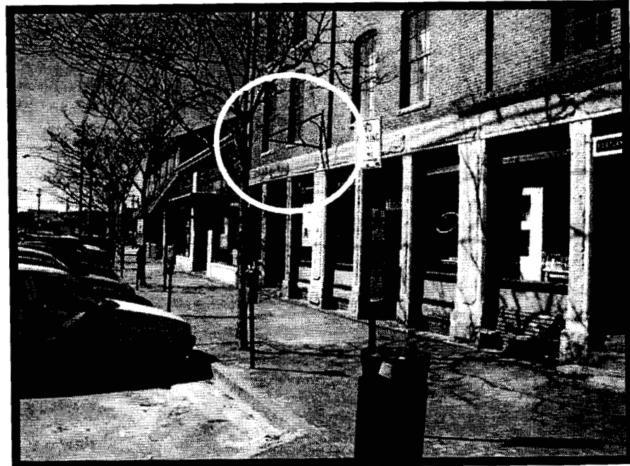
Existing Sign Bracket to be used noted in circle
