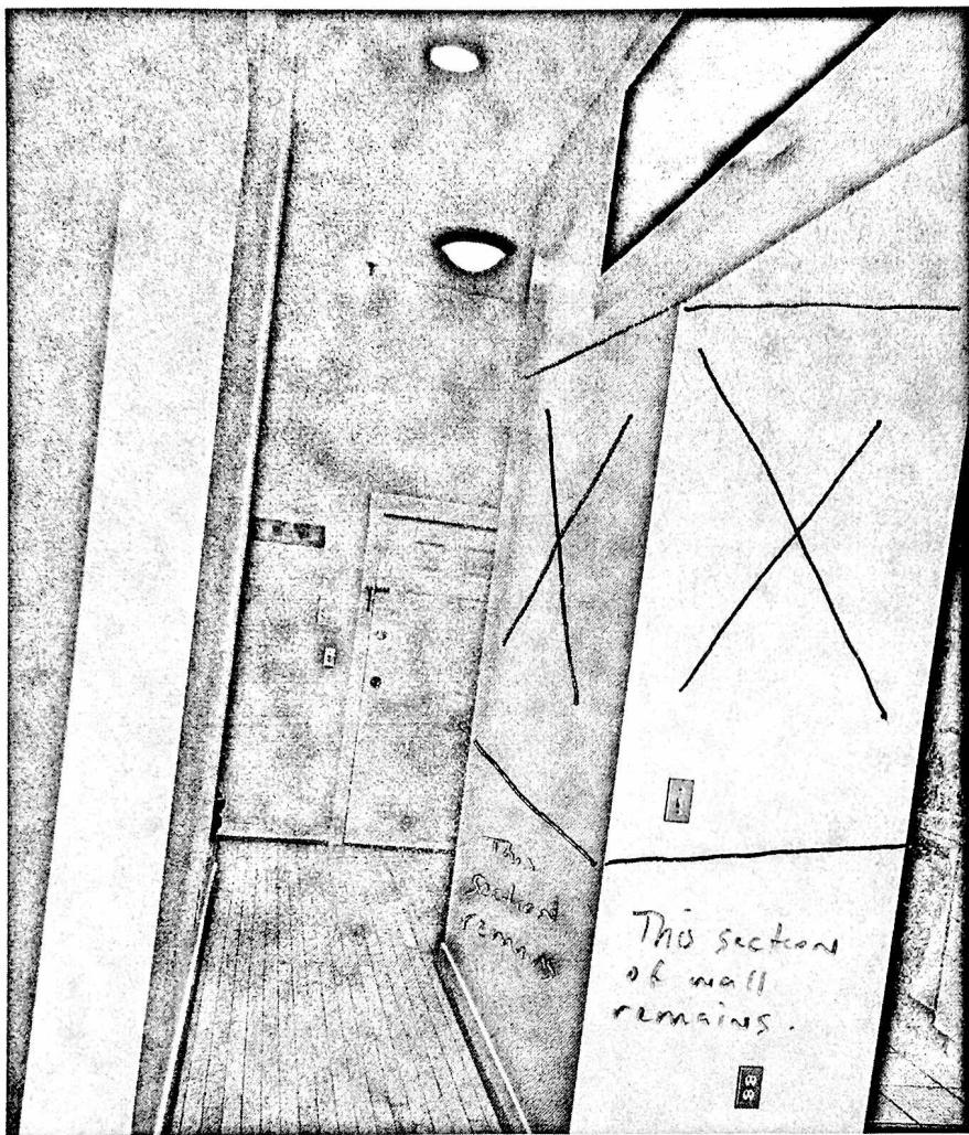
I am enclosing image "A" and "B" to provide a depiction of the work to be done. On the images, I have marked the section of the wall that will be removed with an "X". Please note that only a small section of the wall will be removed. Only non load bearing sections of the wall will be removed. There will be no impact on ingress and/or egress to the apartment. No sprinkler systems will be impacted. Thank you.
