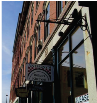
TYPICAL BLADE SIGNS AT SITE
