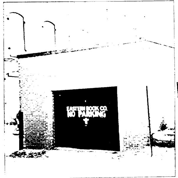
Front of Bldg. 131 Middle St
