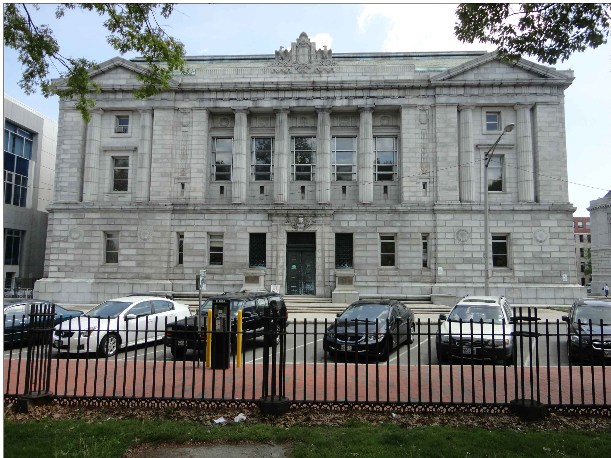
FEDERAL STREET FACADE
