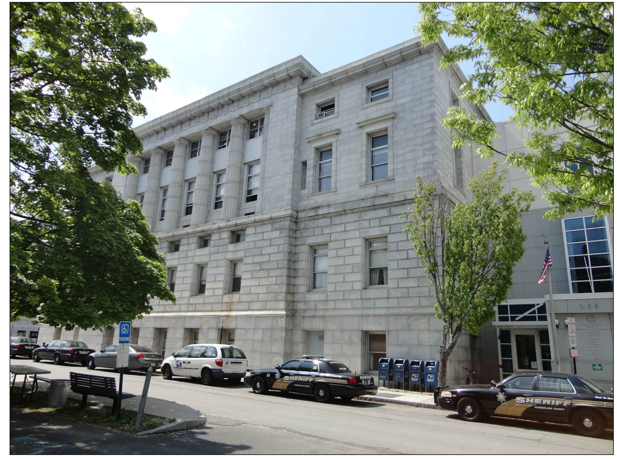
NEWBURY STREET @ CONNECTION TO NEW ADDITION
