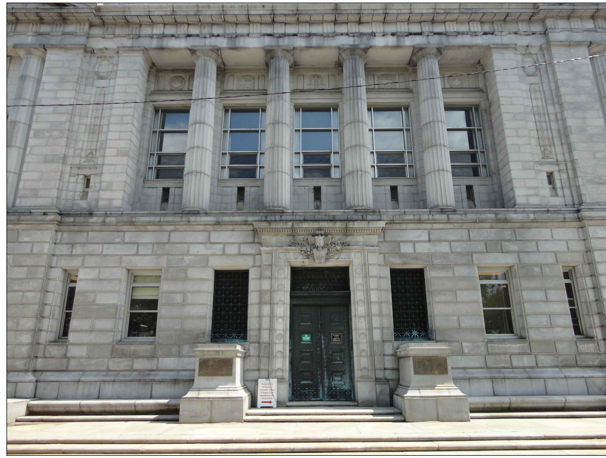
FEDERAL STREET - MAIN ENTRY
