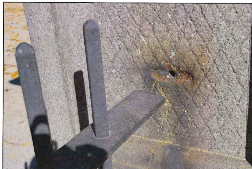
TYPICAL UPPER RAIL - NEW ANCHOR METHOD
