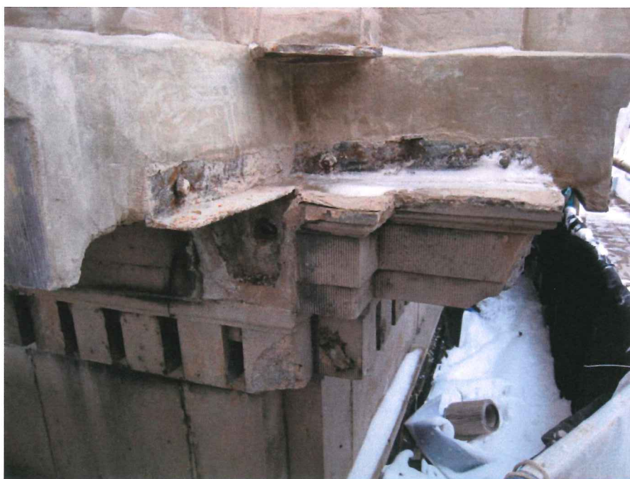
Upper cornice SE corner units removed and patched. MWA 1.5.10
