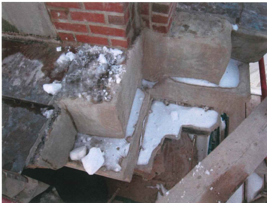
Upper cornice NE corner units removed and patched. MWA 1.5.10
