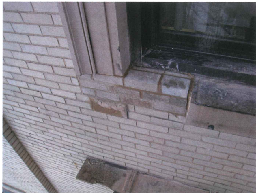
Window sill partial removal and temporary replacement with brick. MWA 1.5.10
