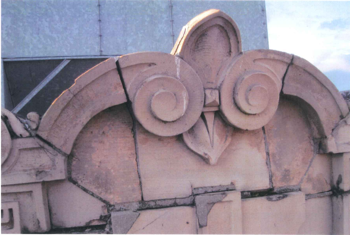
Photo 13: Detail of parapet cartouche. Structures North, Dec 2009.
