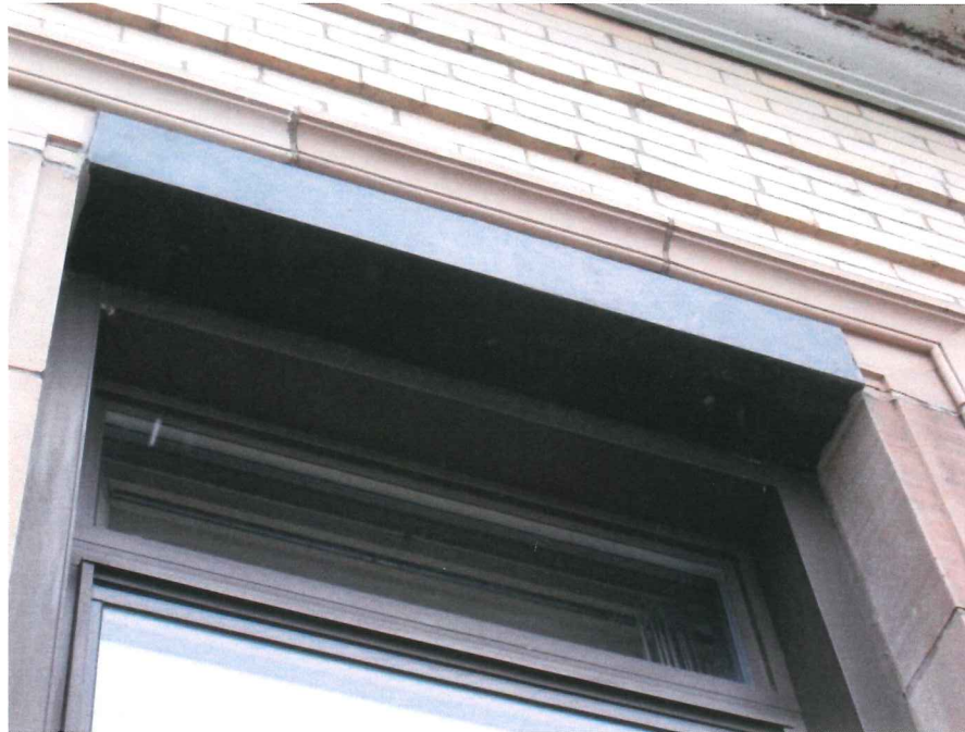
Window lintel soffit stabilization with metal angle. MWA 1.5.10
