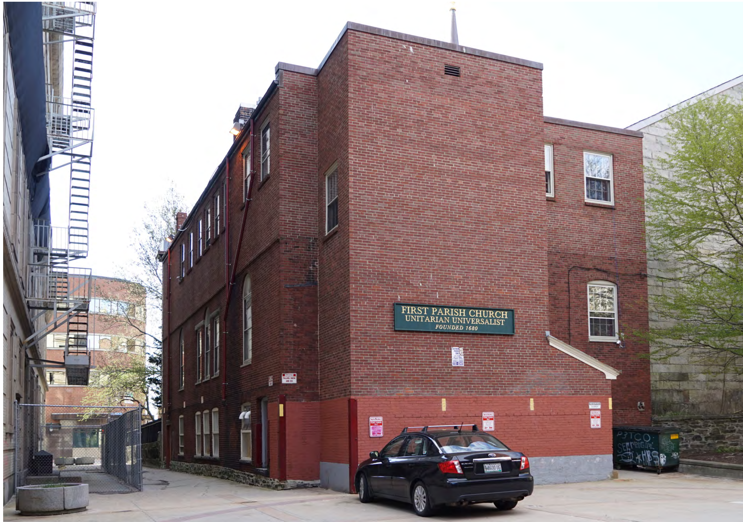
View of Freshman Alley and the rear of the Parish House looking south. The egress stair tower will be removed and replaced with a stair tower, elevator, vestibule and canopy in Phase II.
