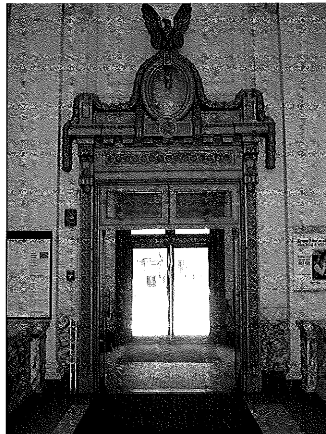
A3 PHOTO - INTERIOR LOOKING TOWARD ENTRYWAY
