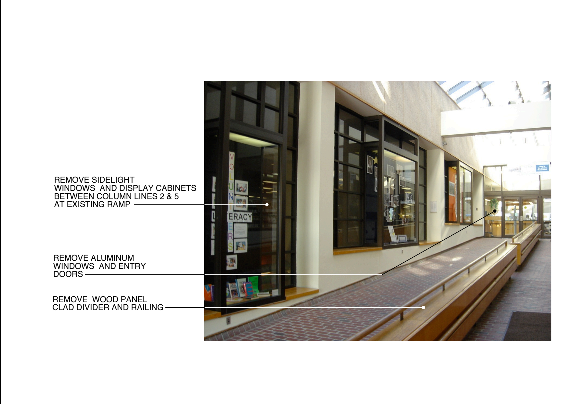
3 DEMO PHOTO, EXISTING ENTRY RAMP NTS
