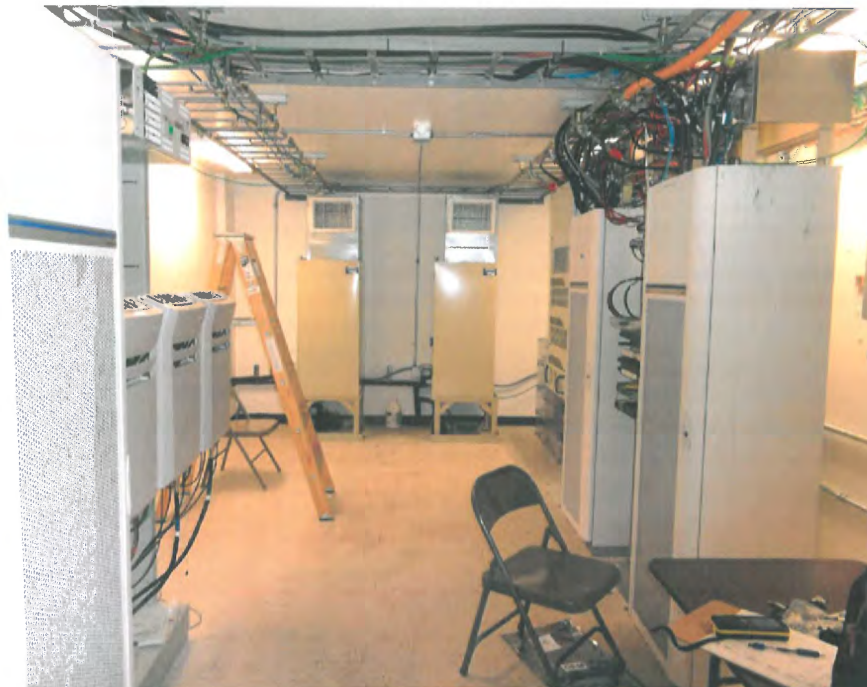
Photo 4: Sample photo illustrating the existing equipment.
