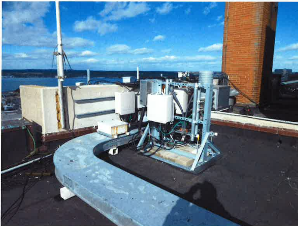
Photo 4: Sample photo illustrating the existing Gamma sector RRH's.
