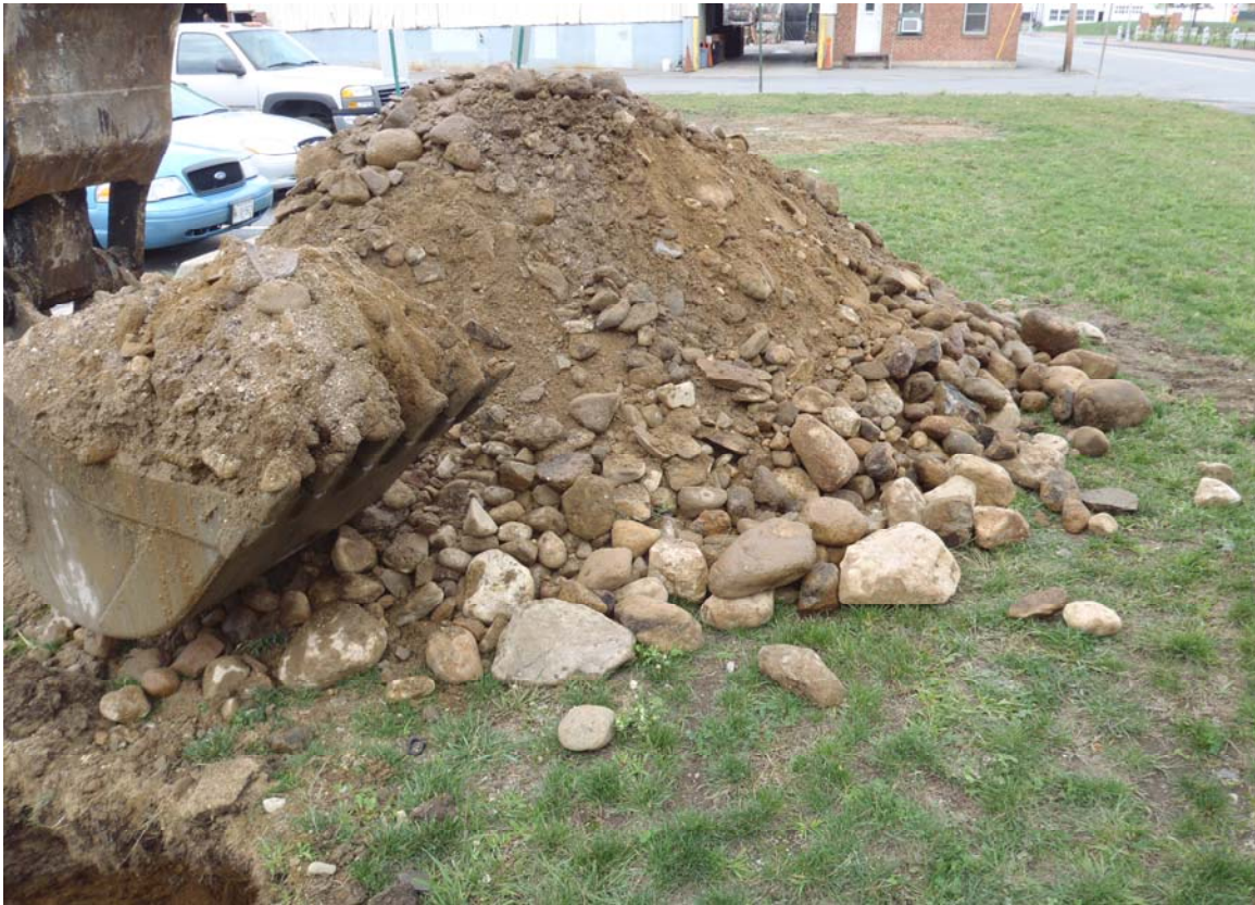
Test Pit TP-2
