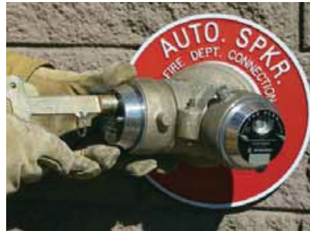
Locking 2 1/2" Plug with Knox Keywrench
