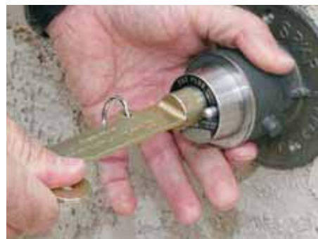
Locking 1 1/2" FDC Plug with Knox Keywrench
