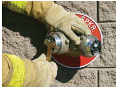
Loosening 2 1/2" Plug with Knox Keywrench
