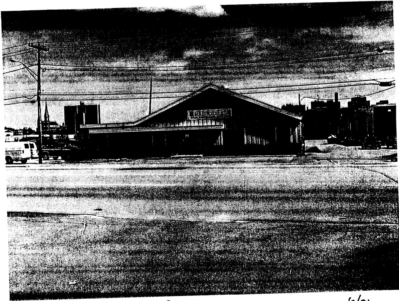
135 MARGINAL WAY - PORTLAND, MAINE DEMOLITION PERMIT PHOTOGRAPH
