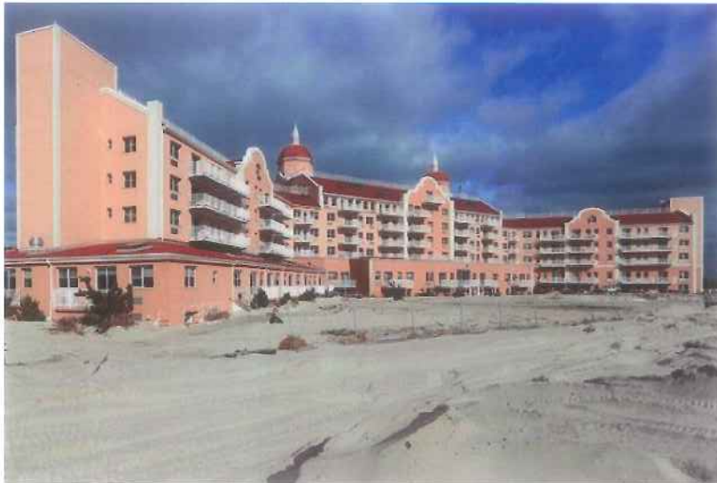
The Lido Beach Towers on Long Beach Island in New York, a structure that was re-clad in EIFS, survived Superstorm Sandy intact, despite the devastation of the property and the interiors.
