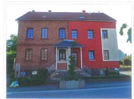
A historic brick building in Germany covered with EIFS on the right side.
