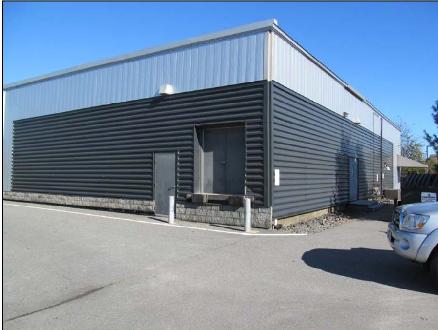
PHOTO 21 – AT&T Store & Planet Dog Building (Year Built 1981)
