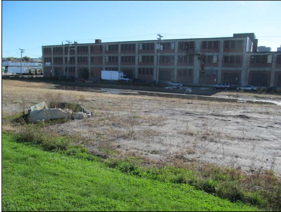
PHOTO 3 – Three Story Concrete Masonry Building (currently storage) (Year Built 1925)
