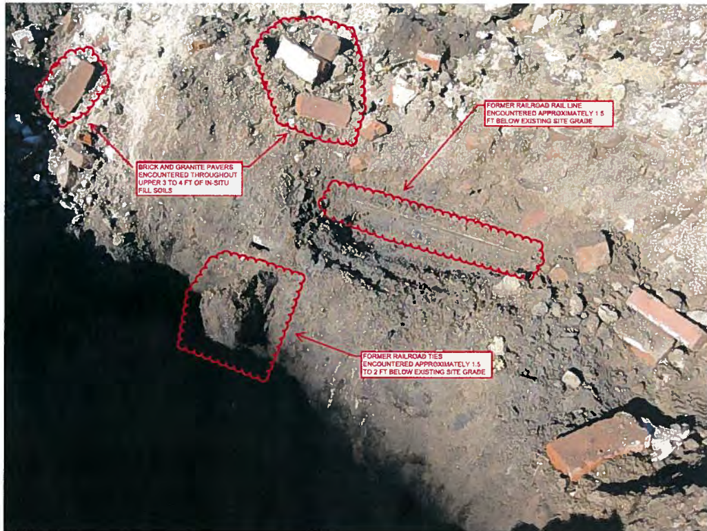
Photograph 1. In-situ fill soils encountered in TP-201, looking northwest (10/20/08).
