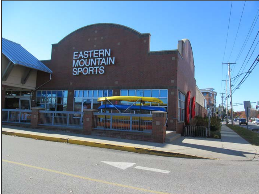
PHOTO 1 – Trader Joe’s & Eastern Mountain Sports Building (Year Built 2001)
