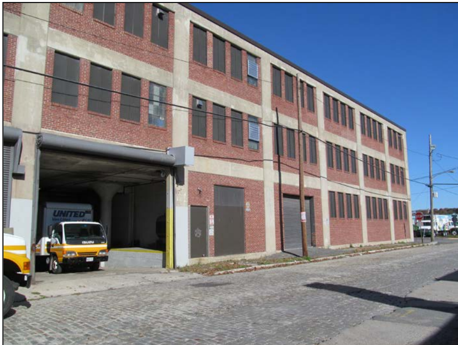
PHOTO 6 – Three Story Concrete Masonry Building (currently storage) (Year Built 1925)
