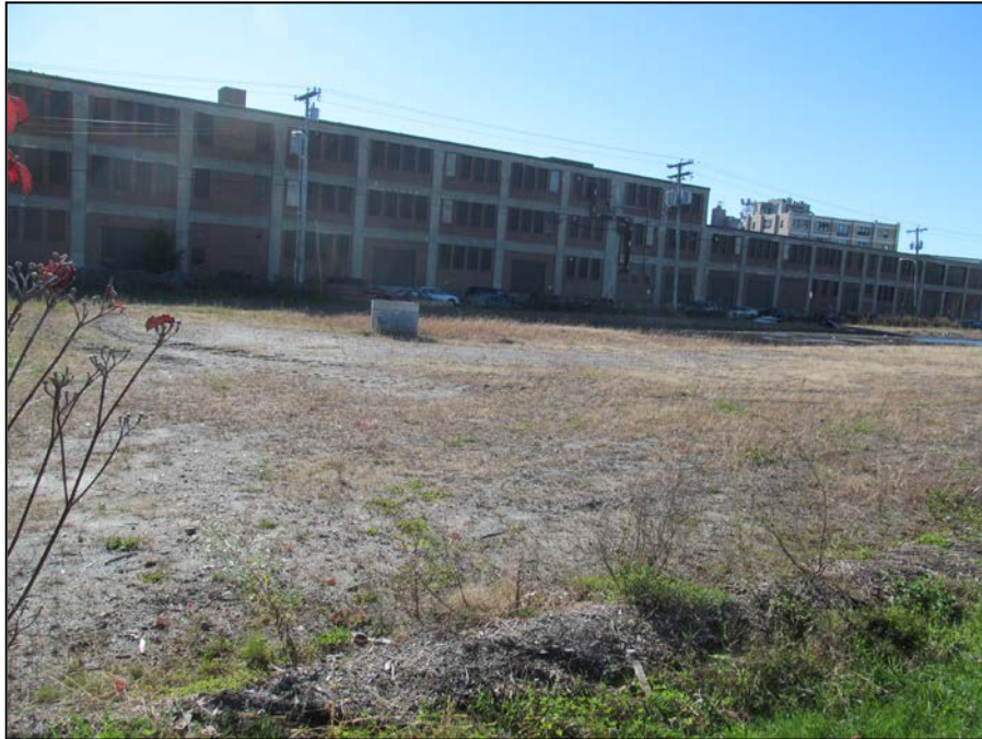
PHOTO 5 – Three Story Concrete Masonry Building (currently storage) (Year Built 1925)
