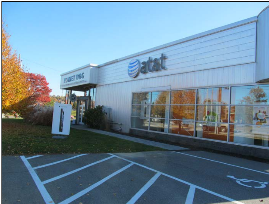
PHOTO 22 – AT&T Store & Planet Dog Building (Year Built 1981)
