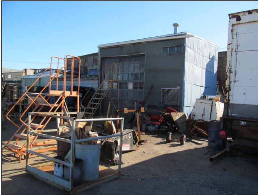
PHOTO 17 – Warehouse Construction Yard Area (Year Built 1940)
