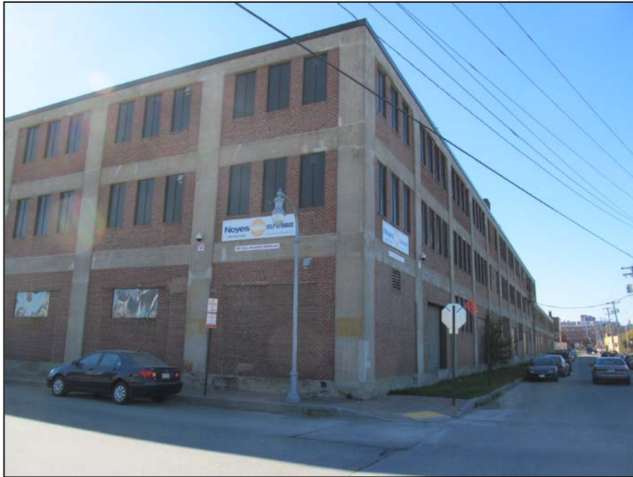
PHOTO 12 – Three Story Concrete Masonry Building (currently storage) (Year Built 1925)
