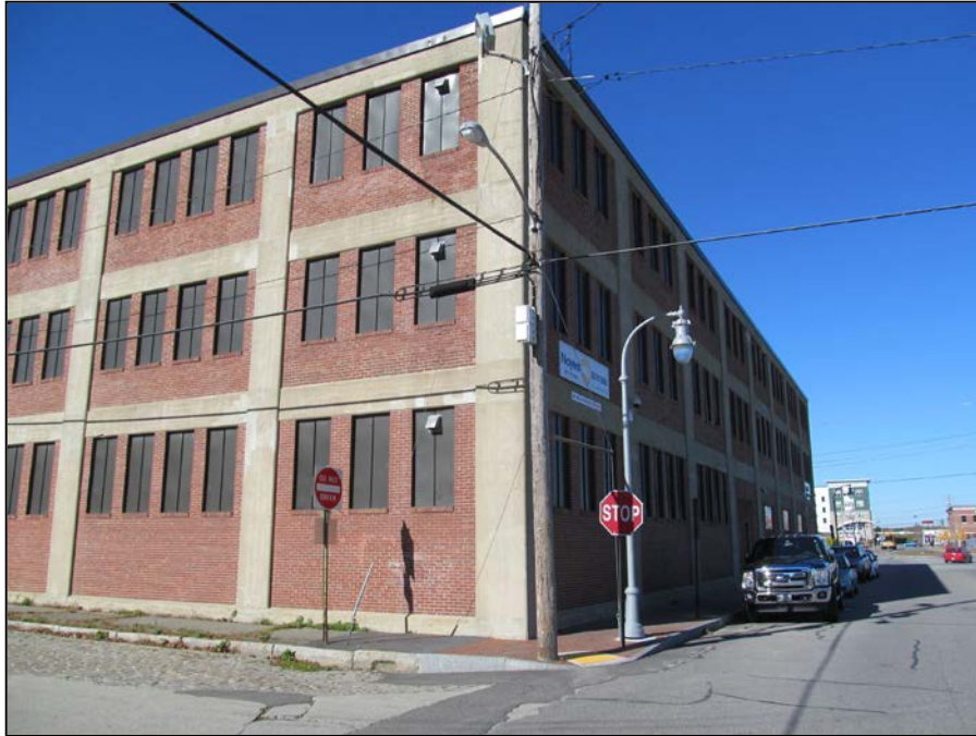
PHOTO 13 – Three Story Concrete Masonry Building (currently storage) (Year Built 1925)
