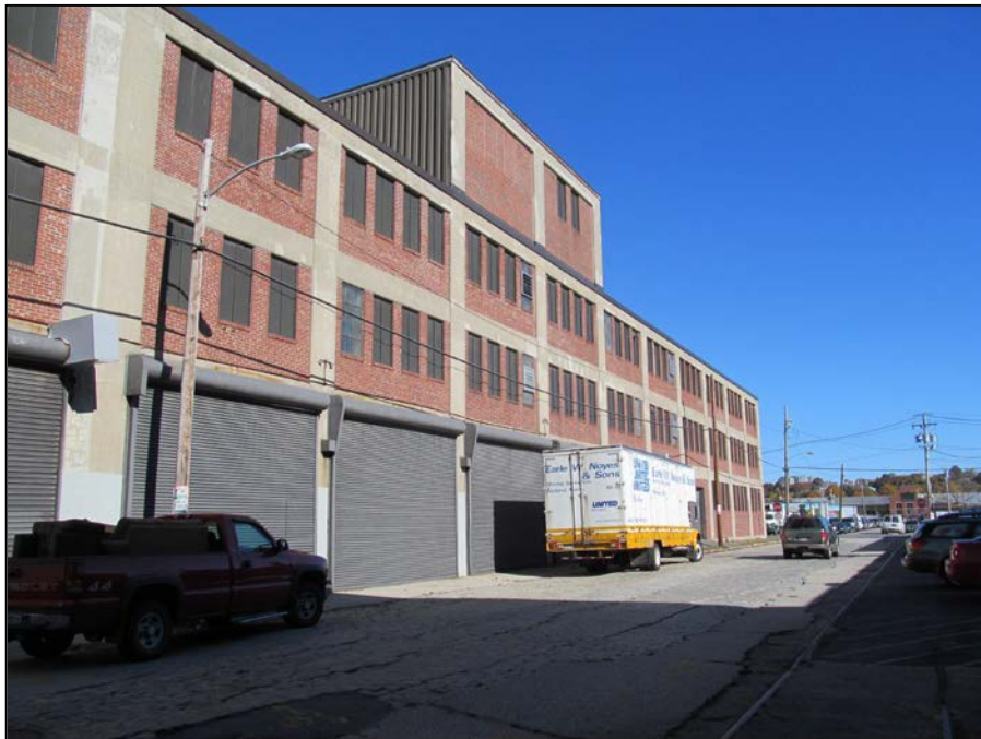
PHOTO 4 – Three Story Concrete Masonry Building (currently storage) (Year Built 1925)
