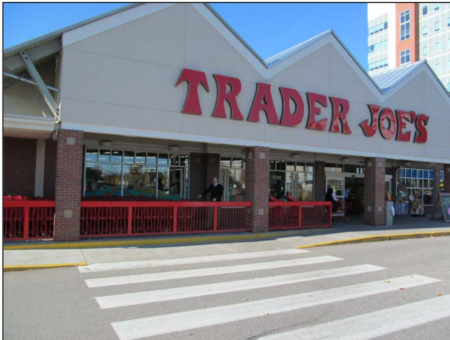
PHOTO 2 – Trader Joe’s & Eastern Mountain Sports Building (Year Built 2001)
