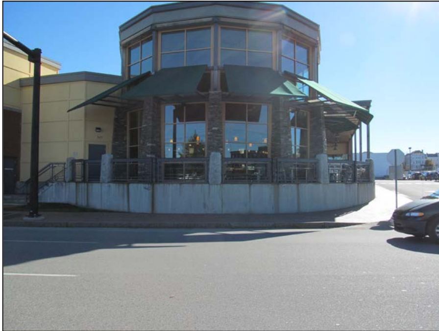
PHOTO 23 – Whole Foods Building (Year Built 2006)
