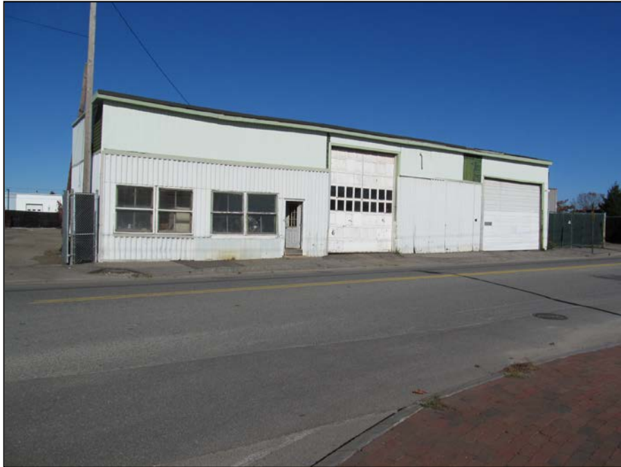
PHOTO 19 – Warehouse Construction Yard Area (Year Built 1940)
