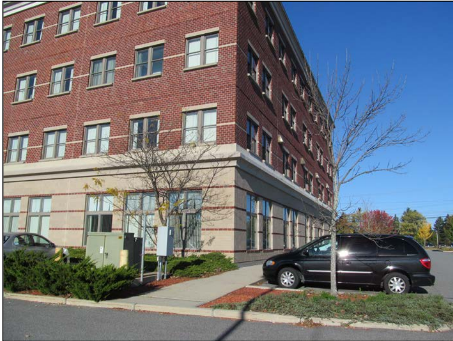
PHOTO 15 – Department of Health & Human Services Building (Year Built 1999)
