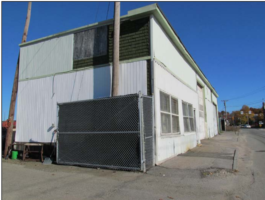
PHOTO 18 – Warehouse Construction Yard Area (Year Built 1940)
