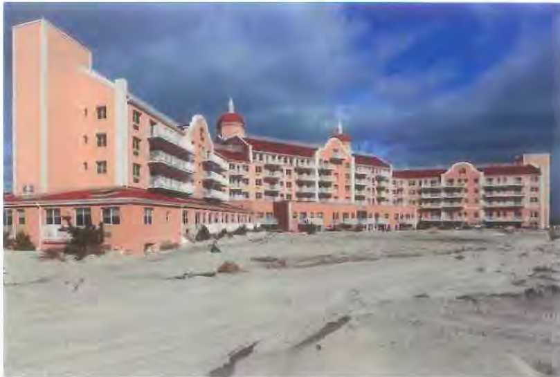
The Lido Beach Towers on Long Beach Island in New York, a structure that was re-clad in EIFS, survived Superstorm Sandy intact, despite the devastation of the property and the interiors.
