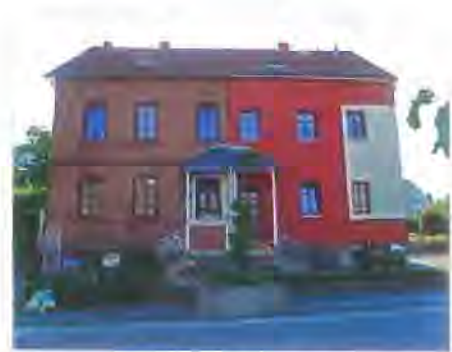
A historic brick building in Germany covered with EIFS on the right side.
