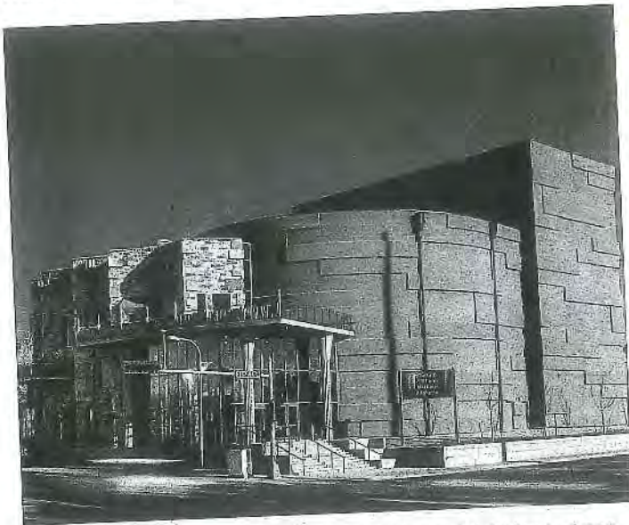
As a lightweight wall cladding, exterior insulation and finishing systems (EIFS) combines insulation with various thin synthetic coatings. Photo courtesy EIFS Industry Members Association
