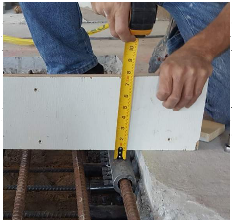
Photo 3: Corrected Coupler w/ Adequate Cover
