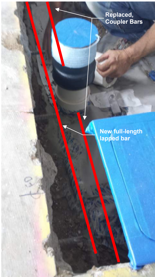
Photo 3: Lapped bars at interfering drain
