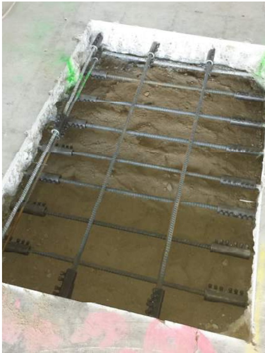
Photo 1: Complete work in opening 1
