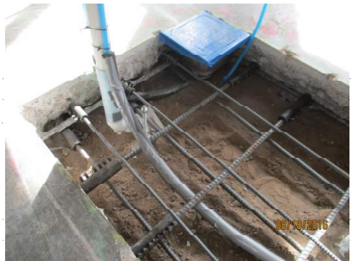
Photo 1: Slab Reinf and Couplers in Opening 5
