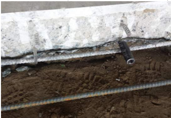
Photo 1: Bars Bent Down to Fit New Coupler
