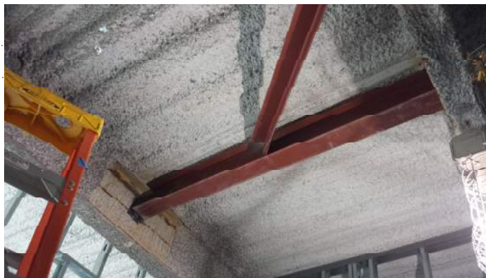
Photo 3: OR Mounting Structure
