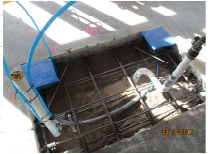
Photo 4: Slab Reinf and Couplers in Opening 5 with Diagonal Dowels Installed
