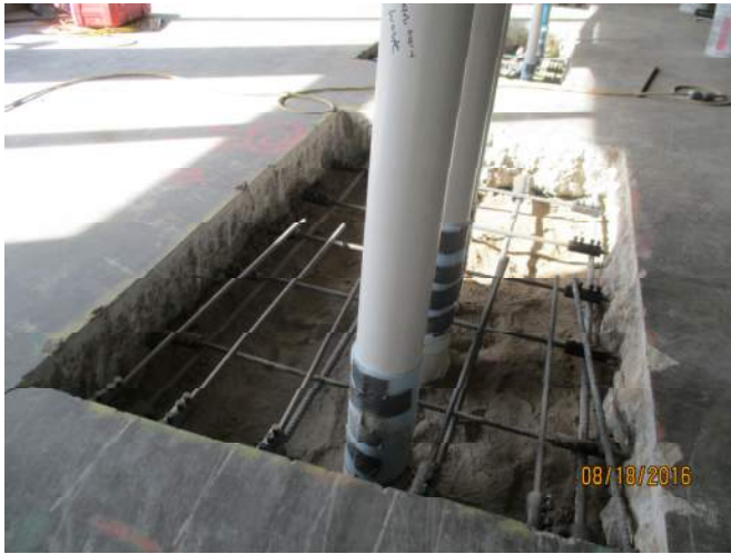
Photo 3: Slab Reinf and Couplers in Opening 4
