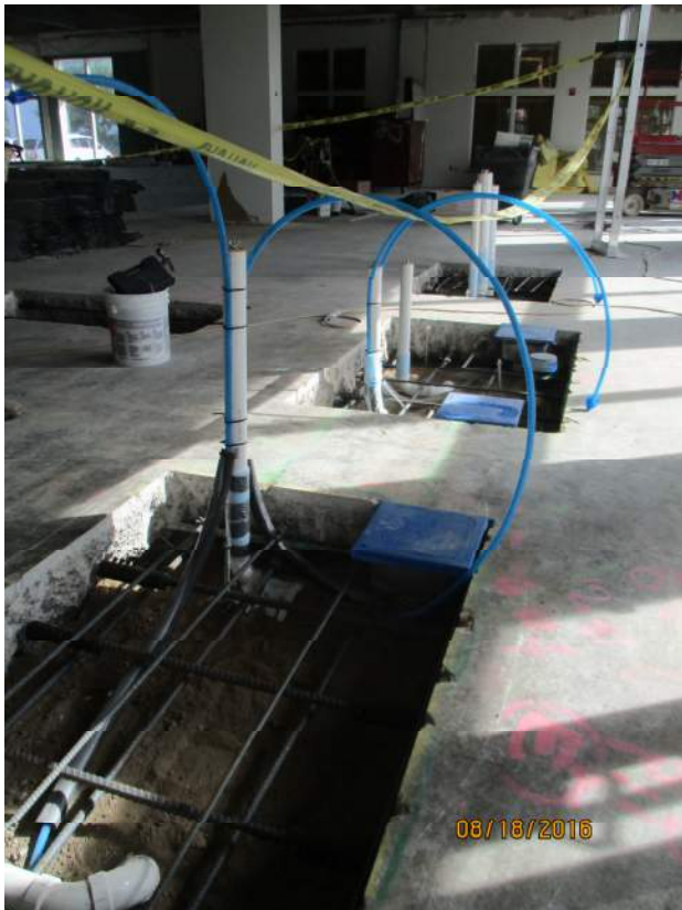
Photo 1: Slab Reinf in Openings 3, 4 and 5
