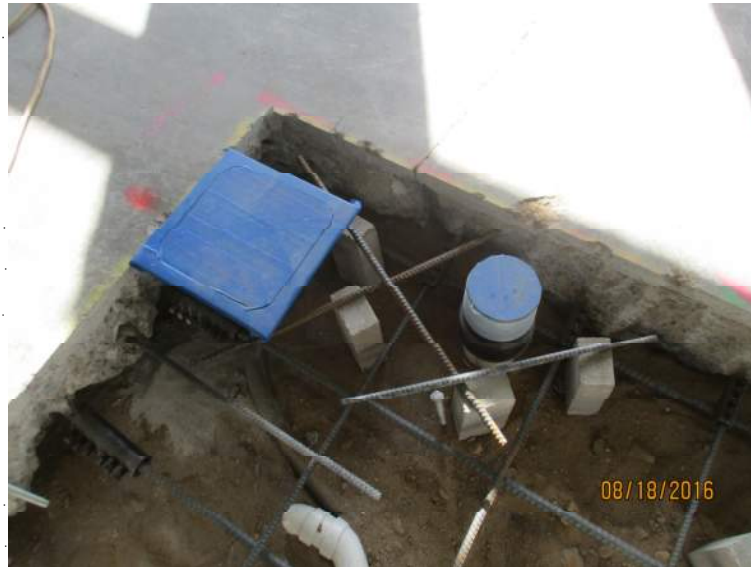
Photo 5: Slab Reinf and Couplers in Opening 3 with Diagonal Dowels Installed
