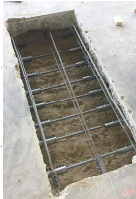
Photo 2: Complete work in opening 2
