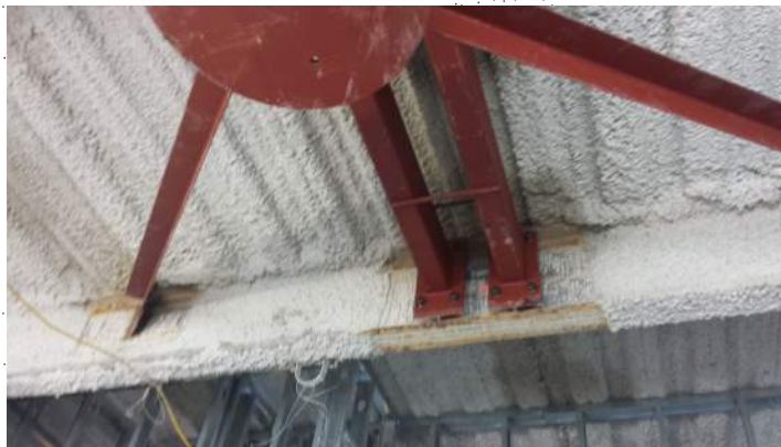
Photo 2: OR Mounting Structure
