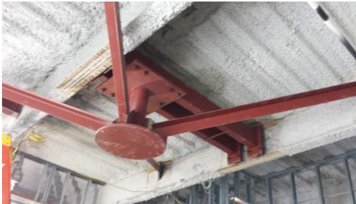
Photo 1: OR Mounting Structure
