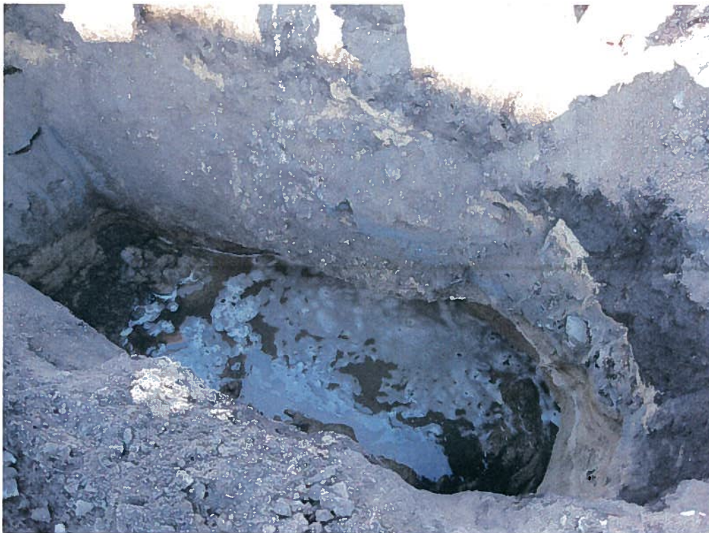
Photograph 2. In-situ fill soils and groundwater encountered in TP-201, looking northwest (10/20/08).
