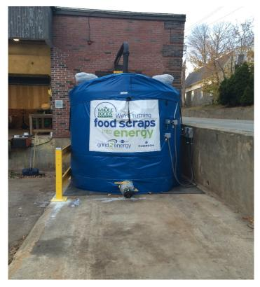
This picture is from the South Weymouth store, and shows the insulated blanket that the tank is covered in to prevent freezing. The bottom center of the tank shows the pipe connect that the pump truck connects to when it gets pumped. This is a very quick process, usually taking no longer than 20 minutes.
