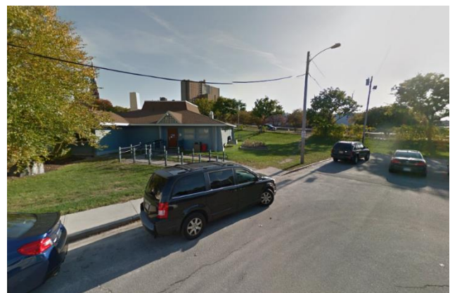
Figure 2: View of Site from Lancaster Street
