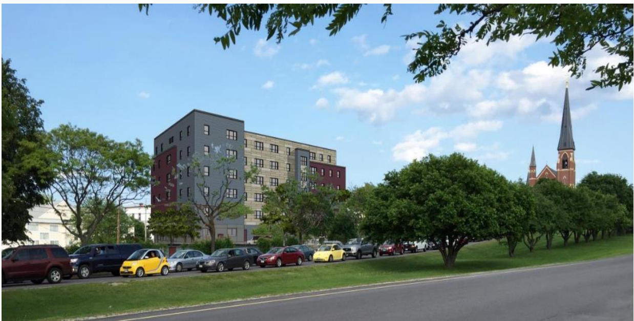
Figure 6: View of the project from Franklin Arterial
