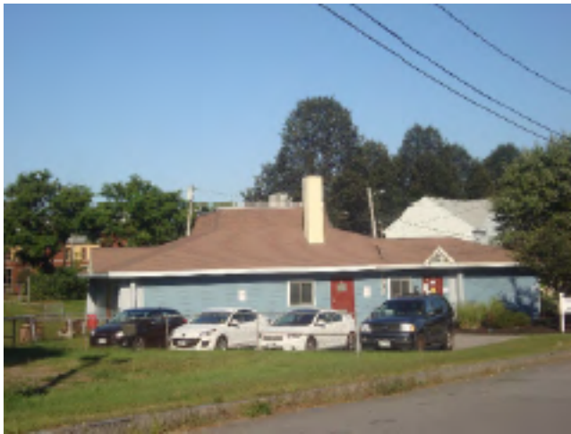
58 Boyd Street existing office building to be demolished. View from Boyd Street.
