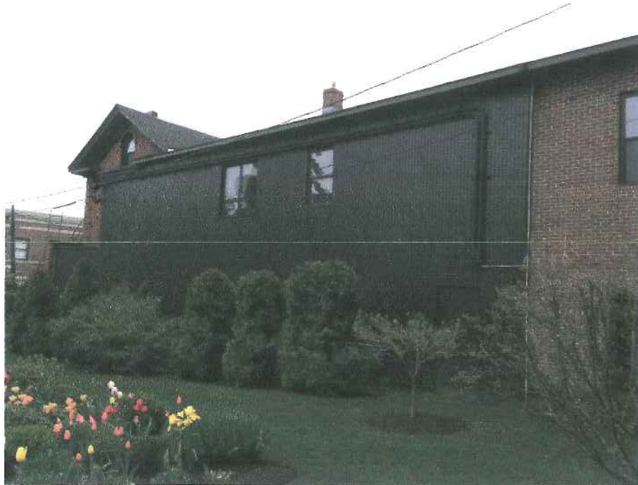
Façade – North Elevation
