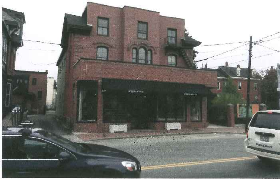
Front (East) Façade
