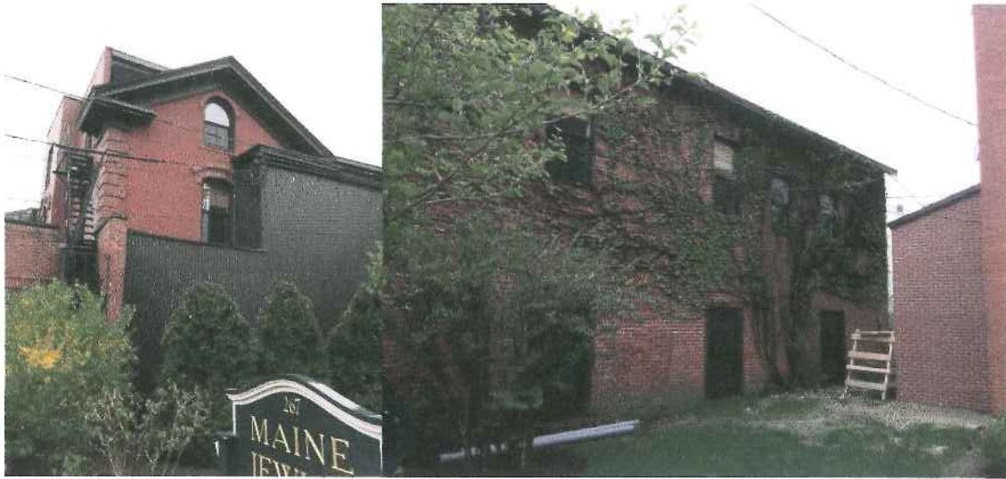
Façade – North Elevation
