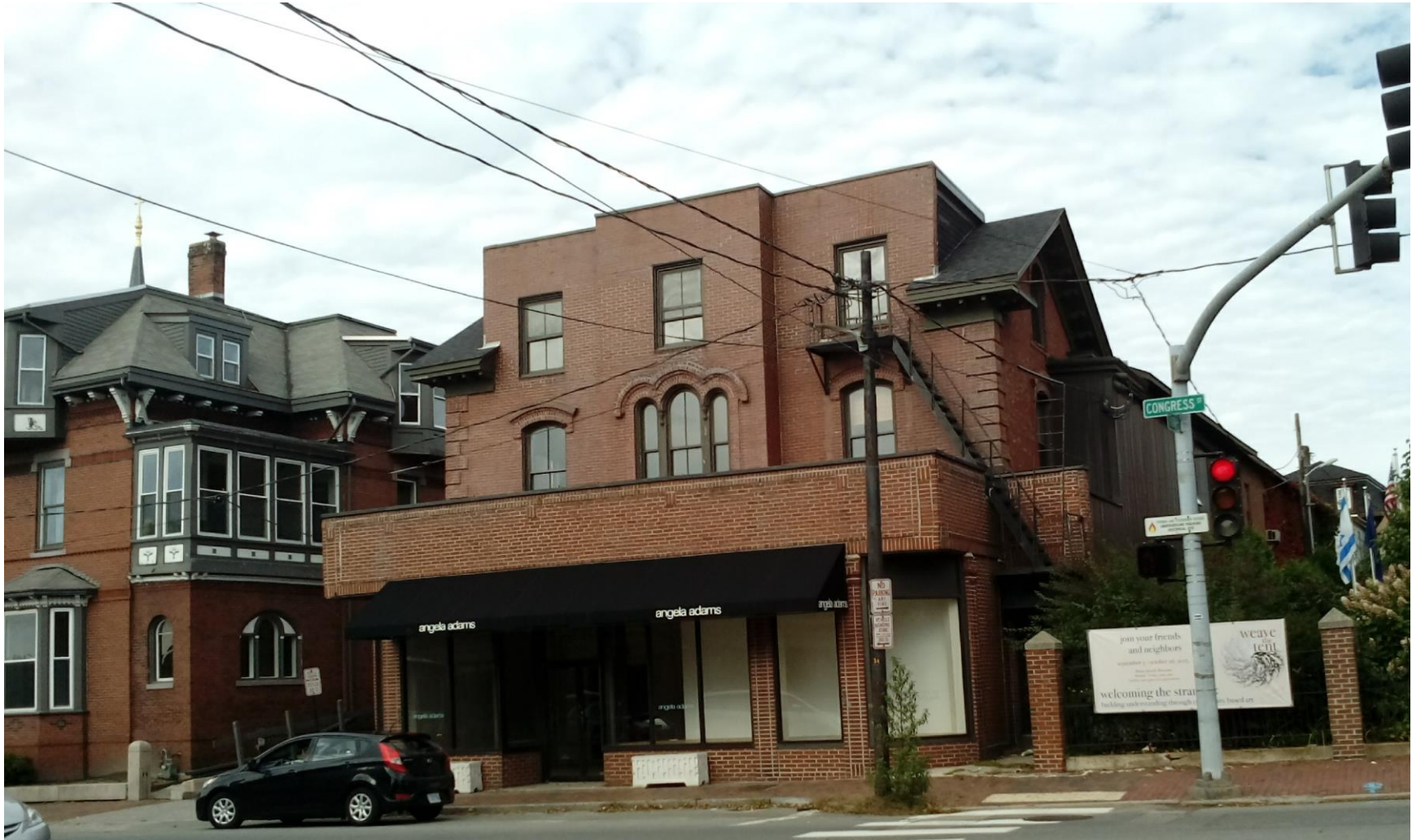
Existing view of front façade
