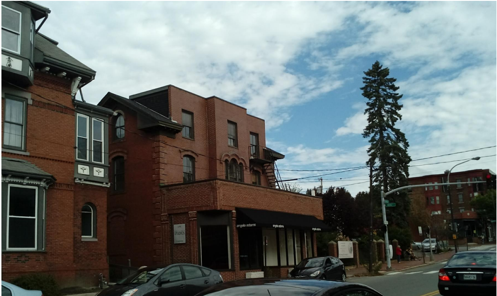
Existing view of front façade
