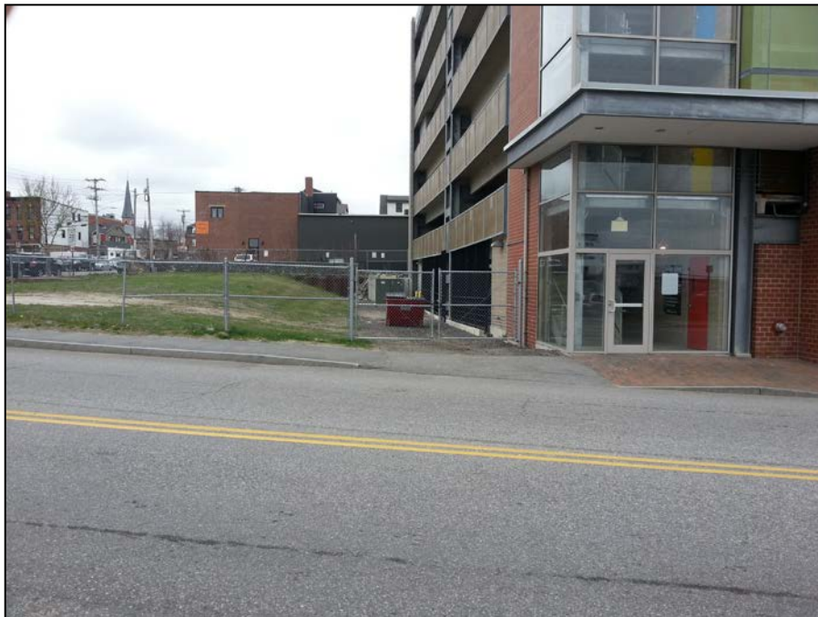
PHOTO 2 – View from Fore Street of shared alley between project site (left) and Ocean Gateway Garage (right)
