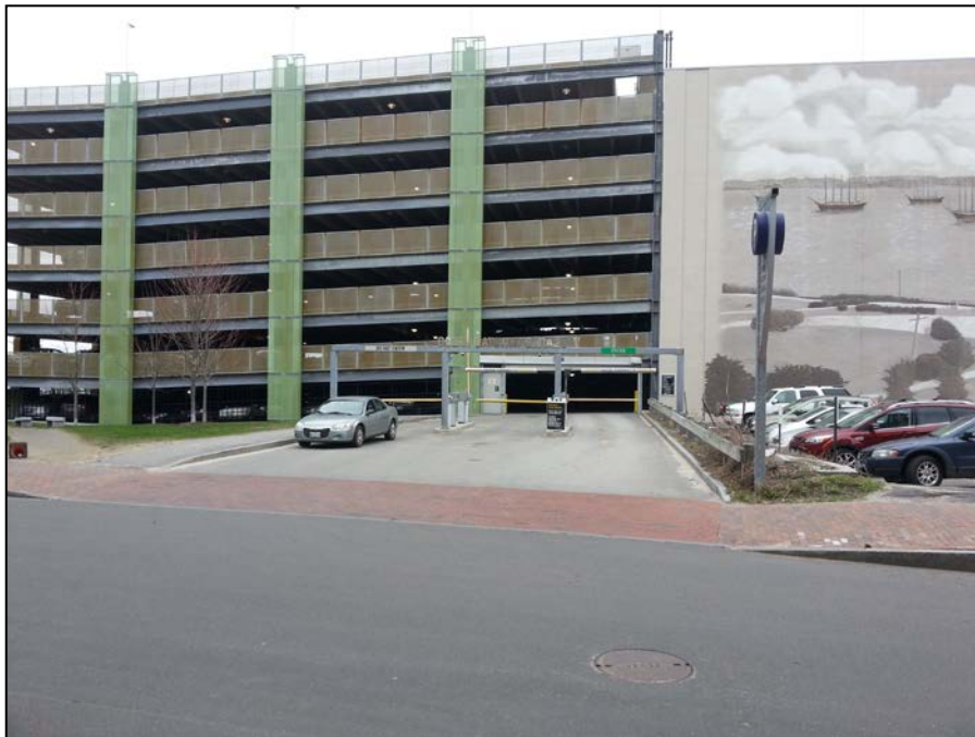
PHOTO 2 – View from Middle Street across the site along entrance drive to Ocean Gateway Garage
