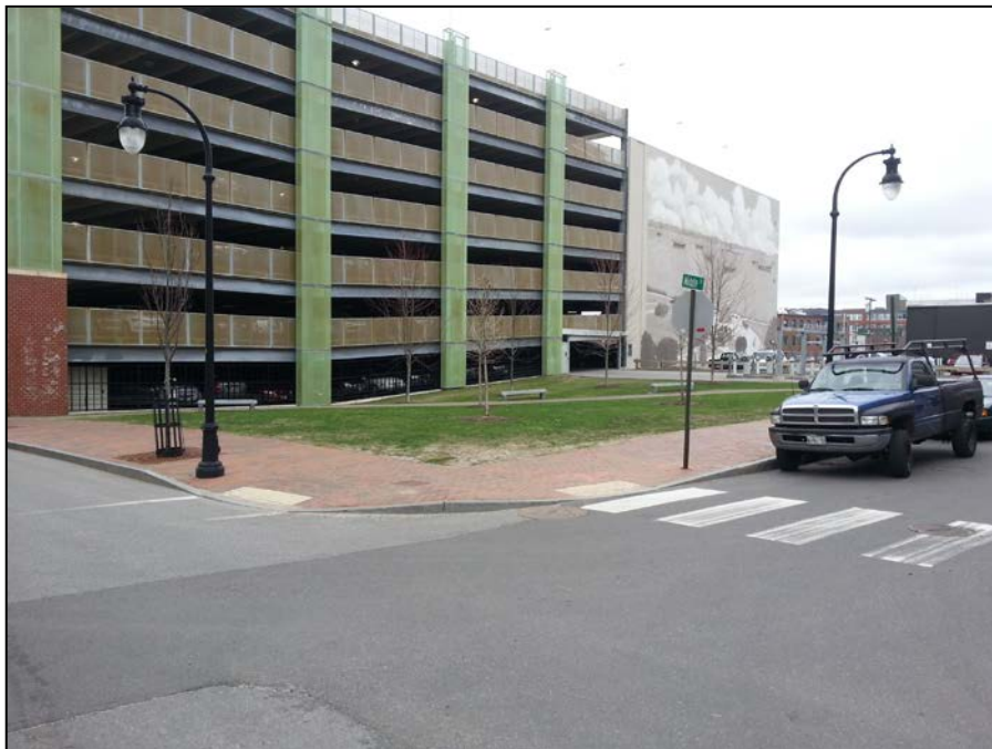
PHOTO 4 – View of site from intersection of Middle Street and Hancock Street Extension
