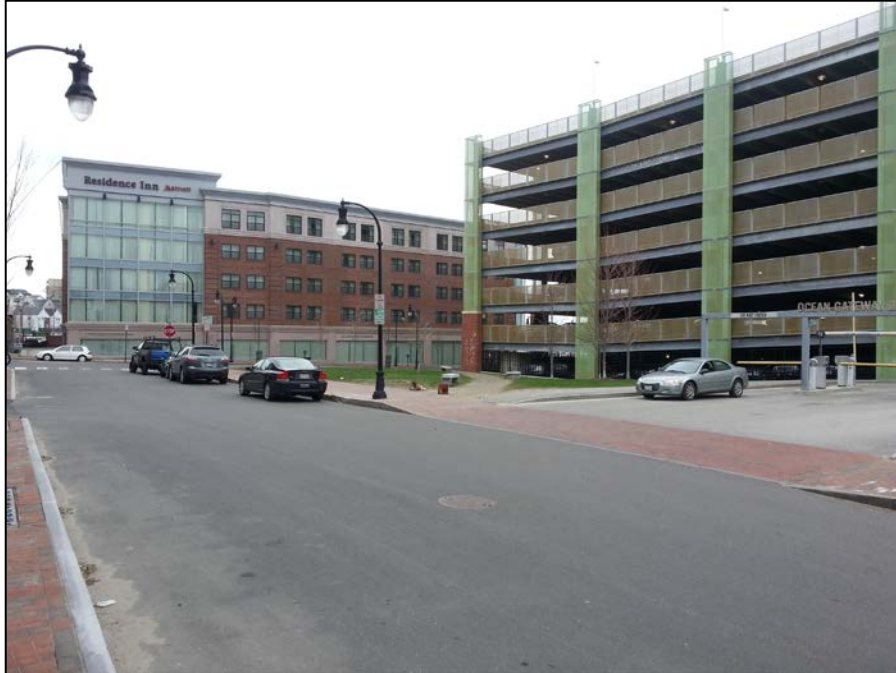
PHOTO 1 – View of the site from Middle Street
