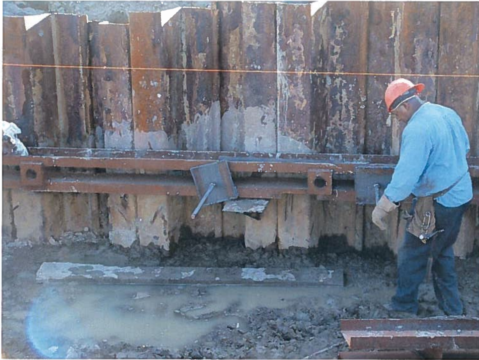
Photograph 5. Tie Back installation at whaler (6/21/07).
