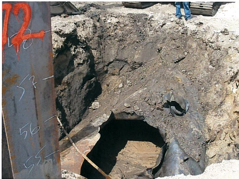
Photograph 10. Excavation at underground tank (6/22/07).
