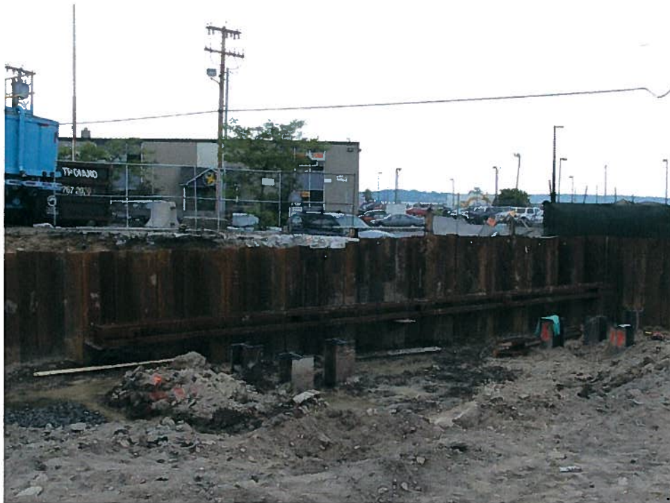
Photograph 4. Whaler installation along sheet pile wall at the elevator pit (6/21/07).
