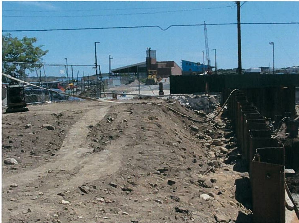
Photograph 8. Fill placed above tie backs and dead man (6/21/07).
