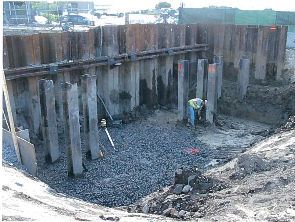
Photograph 9. Excavation at pile caps H-2.3, H-2.7, and H-2.9 (6/22/07).
