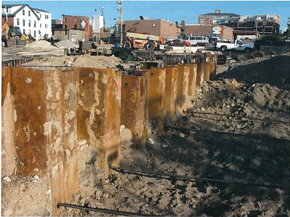
Photograph 7. Tie Backs along sheet pile (6/20/07).
