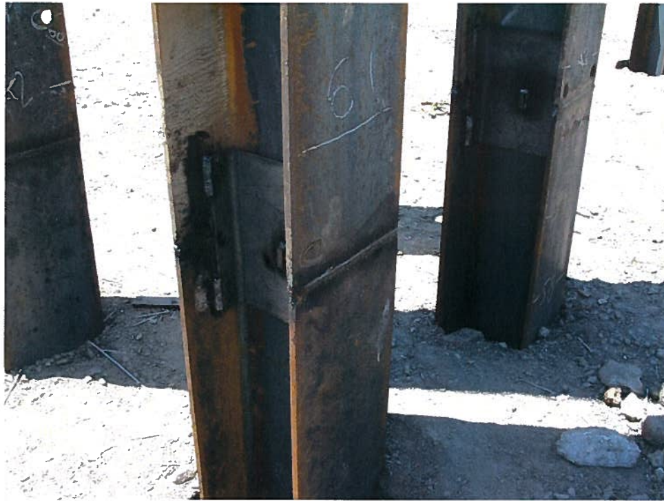
Photograph 3. Typical pile splice with champion connection (6/19/07).
