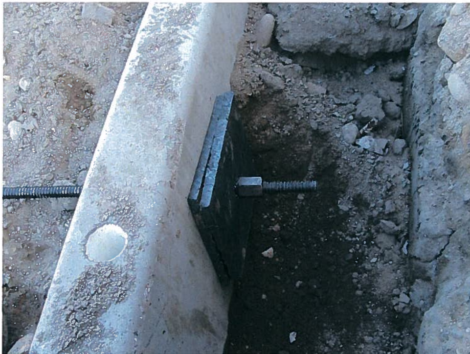
Photograph 6. Tie Back installation at dead man (6/21/07).
