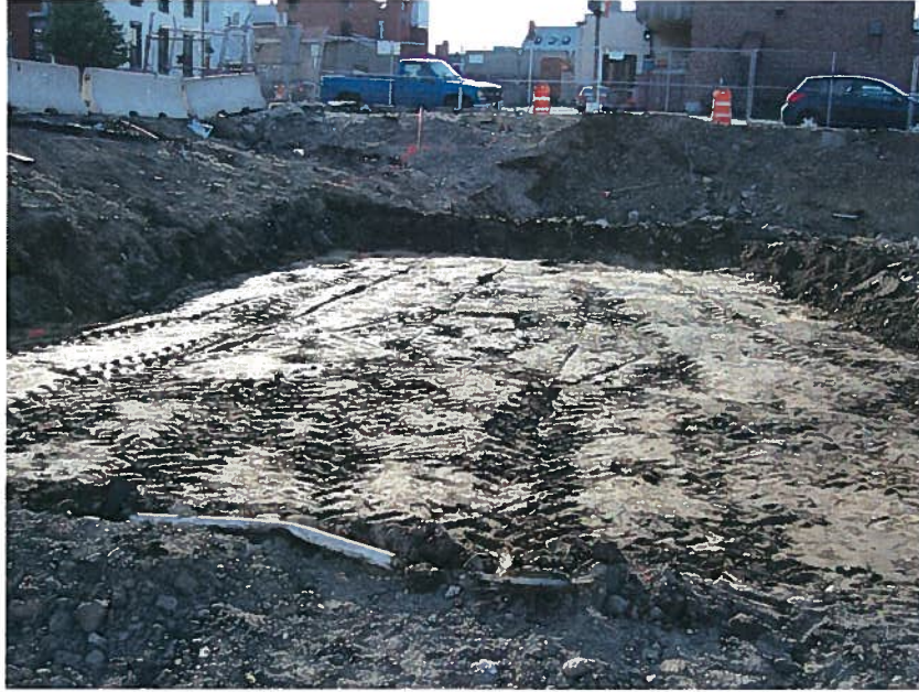
Photograph 3. Prepared subgrade beneath subsurface stormwater chamber, looking west (5/29/07).
