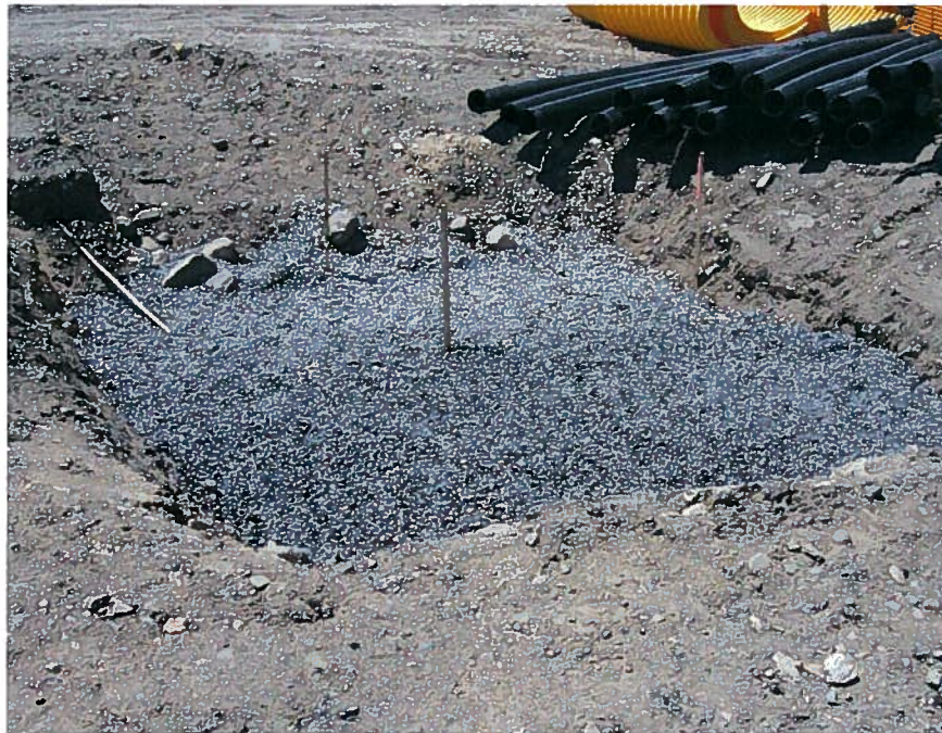
Photograph 2. Crushed stone placed over prepared subgrade at column G-1, looking south (5/29/07).
