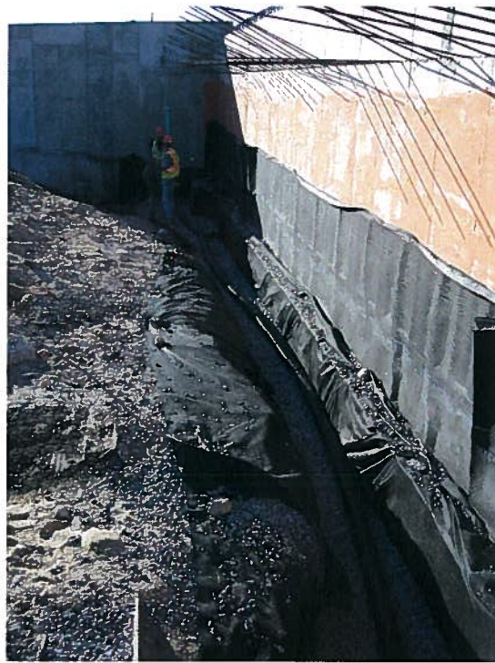
Photograph 3. Installation of underslab drain north of column line D, looking east (8/27/07).
