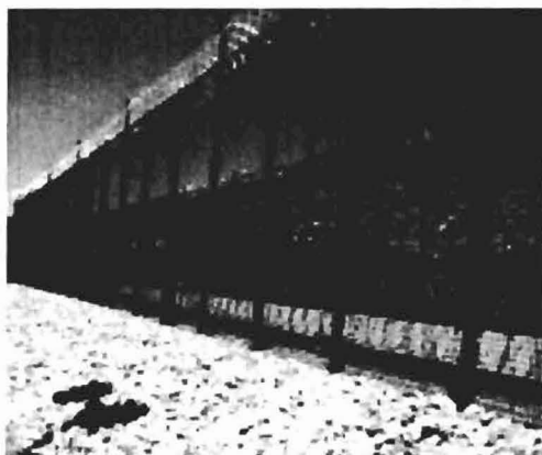
WireWall goes up in panels, saving time and equipment needed for installation.
