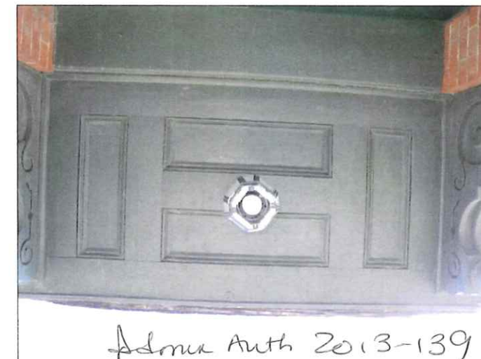
CEILING DETAIL ON ADJACENT PORCH
