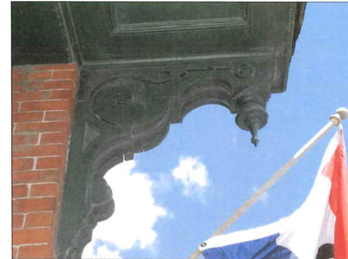
EXISTING DETAILS ON ADJACENT PORCH
