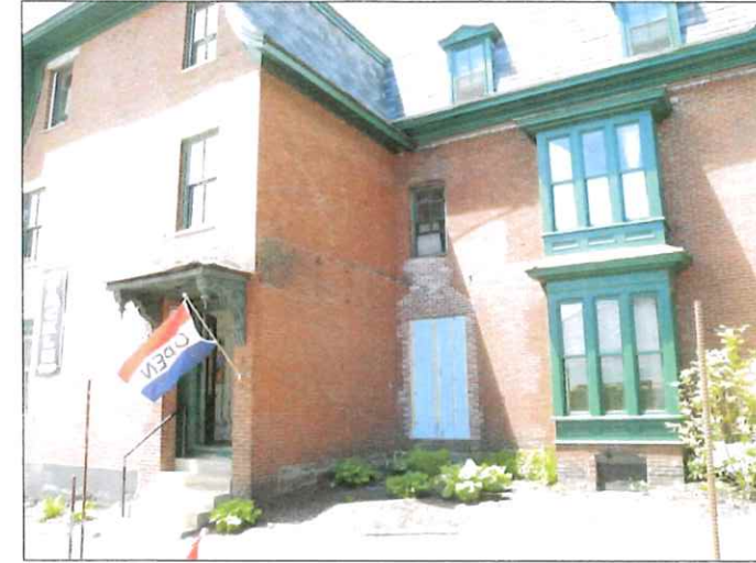
AREA OF WORK AND EXISTING ADJACENT PORCH
